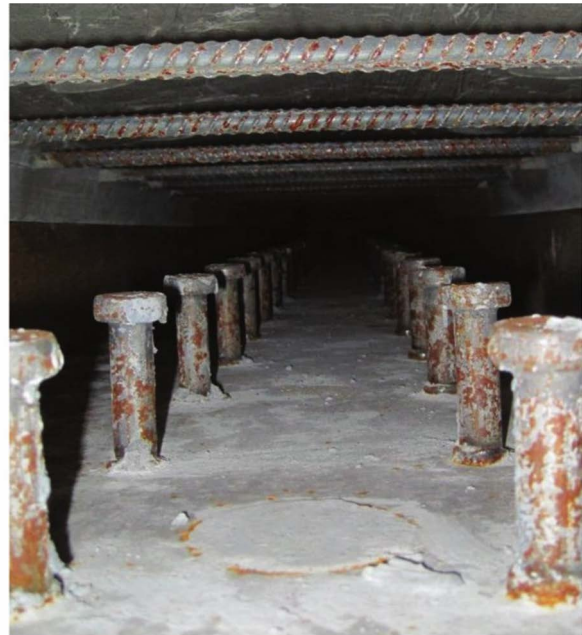
Composite connection detail
