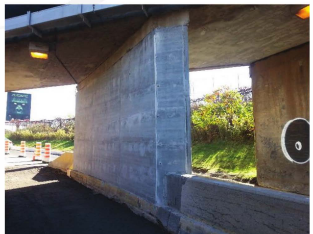
Fig. 6.4—(a) UHPC bridge deck rehabilitation in Switzerland (Brühwiler and Denarié 2013); (b) large-scale structural UHPC deck overlay, Viaduc de Chillon, Switzerland (Brühwiler et al. 2015); and (c) pier repair in Canada (Doiron and Perry 2014).
