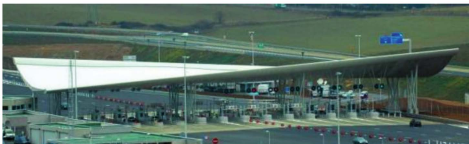
Fig. 6.12b—General overview of Millau Viaduct toll gate roof.
