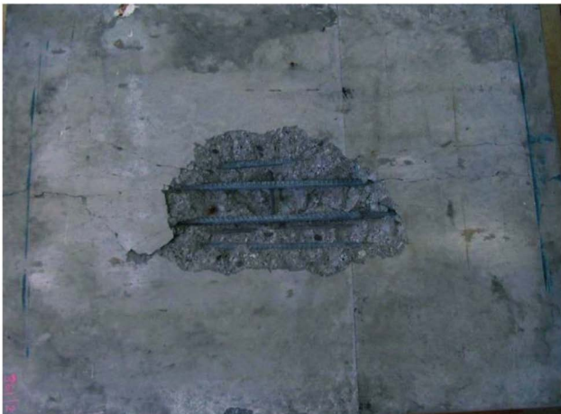
Fig. 6.7b—Back side of 7252 psi (50 MPa) concrete panel (Cavill et al. 2006).
