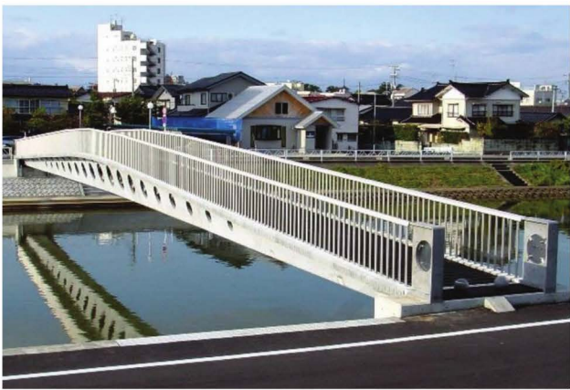
Fig. 6.2b—Sakata-Mirai Bridge (photo courtesy of Lafarge).
