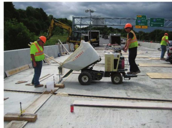
Field casting of UHPC
