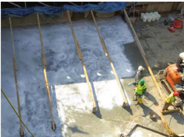
Fig. 6.11c—Placing UHPC in Caderousse Dam Spillway by pump (photo courtesy of Lafarge).
