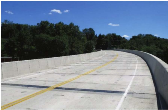
Bridge with UHPC connections
