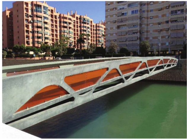
Fig. 6.2d—Pedestrian Bridge over Oveja's ravine, Alicante, Spain (photo courtesy of B. Massicotte).
