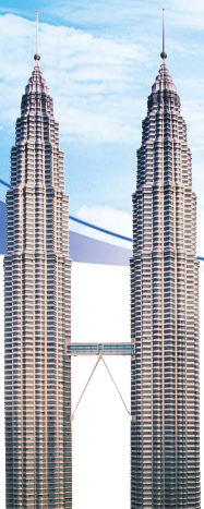
Petronas Towers in Kuala Lumpur, Malaysia Height 451.9m, No. of Floors 92(Plus 6 underground levels) Period 94.3.4- 96.6.16(27 Months)
