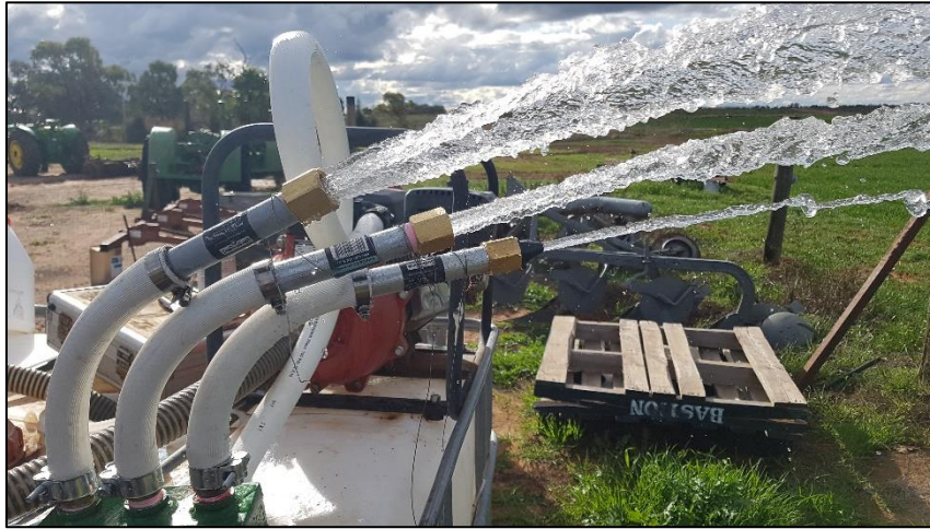
Bench testing the nozzles and manifold using a portable fire fighting unit Showing the flow through a 3/8 (bottom) and 3/4 inch diameter oriface
