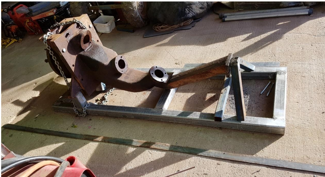
Lining up the nozzle housing during welding
