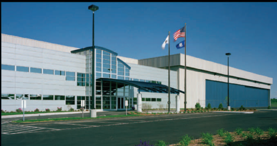
113' W x 29'H, 6-single panel Floating Door Systems
