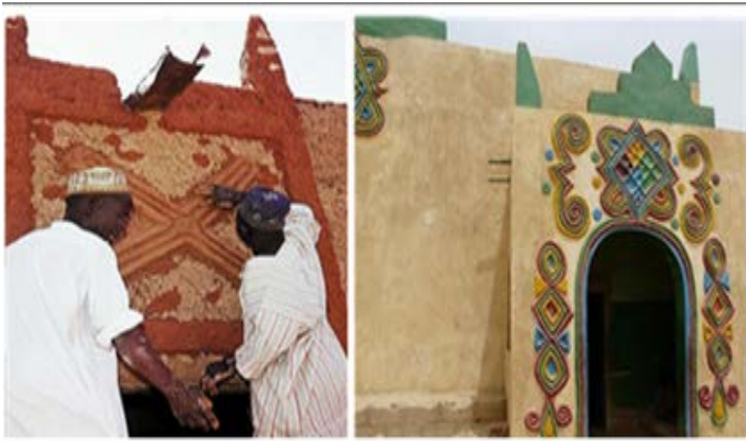
Figure 1: Engraving works (as a unique feature of Vernacular Architecture of Hausa-Fulani in Northern Nigeria)
