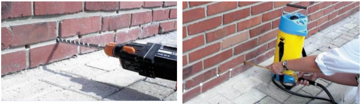
Figure 20. Installation of injectable liquid damp-proofing course (Aida DPC, Remmers Ltd., 2005)
