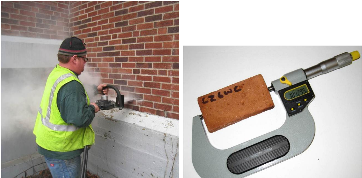
Figure 8. Removal of brick sample, and dilatometry (dimensional change) measurements
