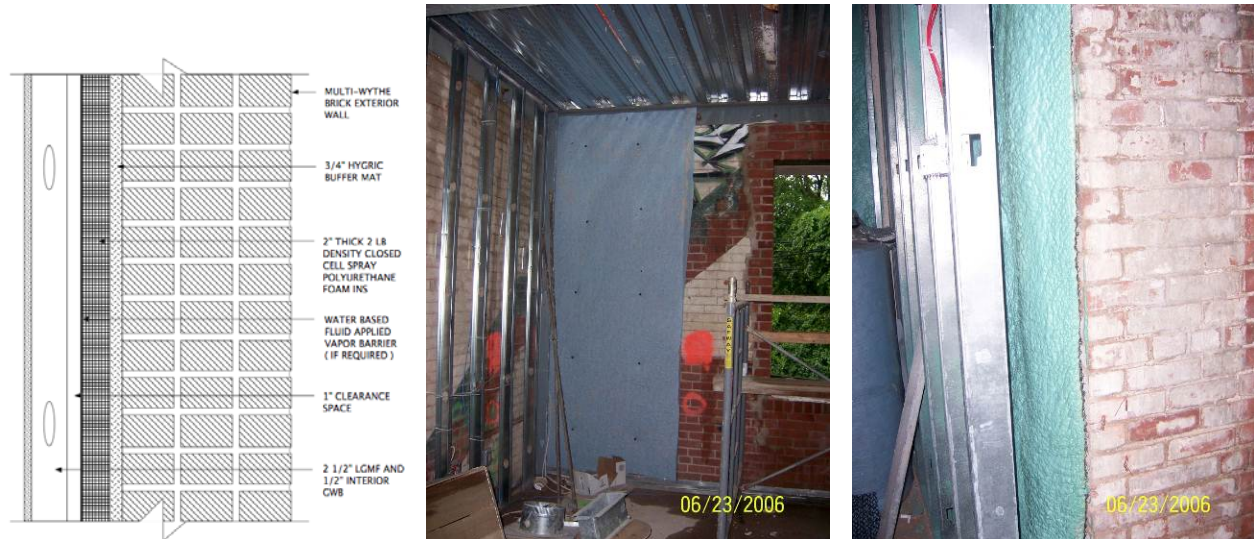
Figure 13. Hygric buffer mat and interior insulation application (Anastasi 2011)
