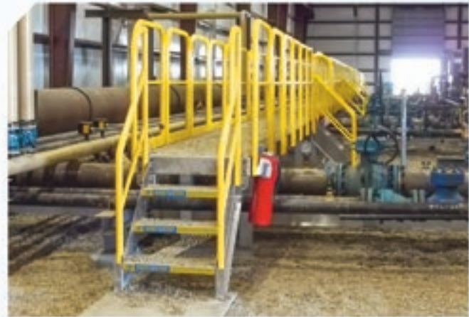
Safely cross numerous different size piping at this gas compressor station.
