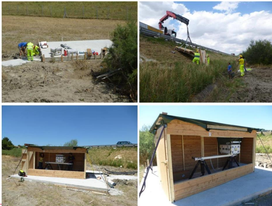
479 Figure 3. Pictures of the construction of the covered structure and installation of the GB-InSAR.
