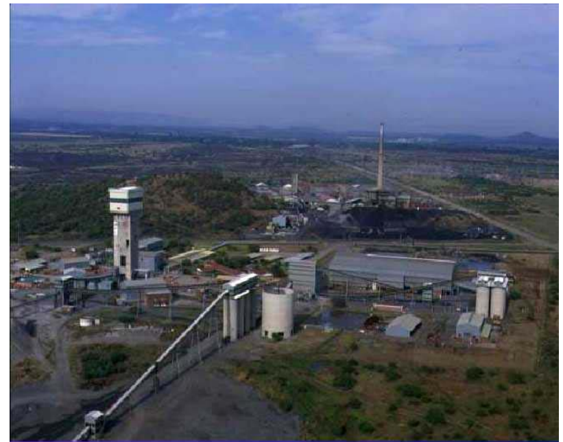
Rowland Shaft, Concentrator, and Smelter
