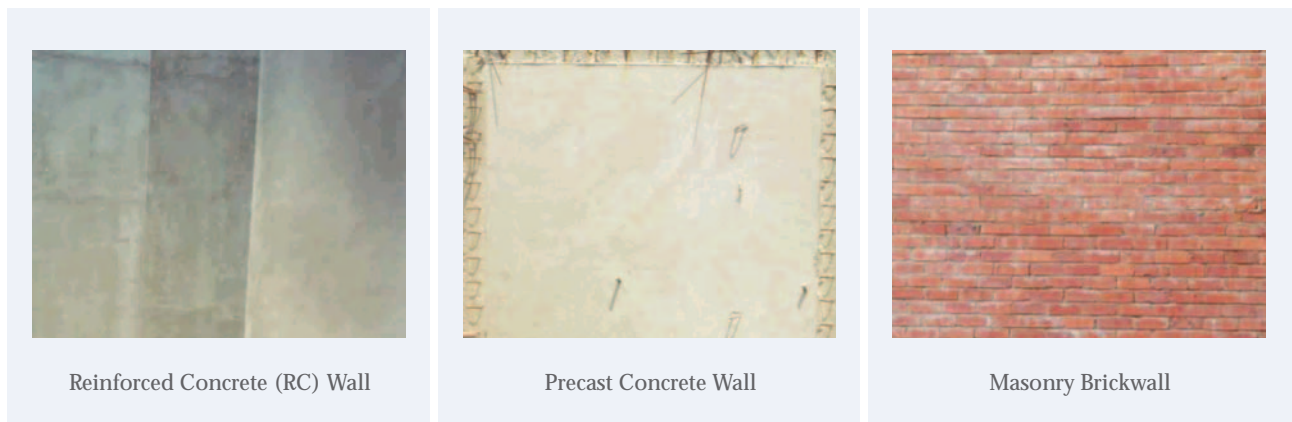
Figure 2.1: Common types of external wall system
