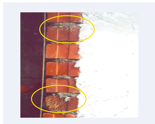
Figure 2.21: Mesh reinforcement embedded at every 4 th course
