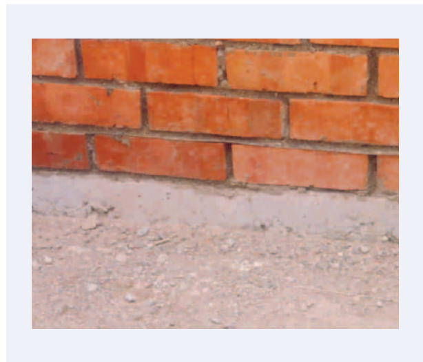
Figure 2.18: Concrete kerb at the base of brickwall
