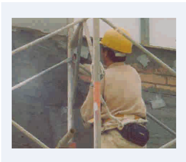
Figure 2.17: Applying rendering to an external brickwall
