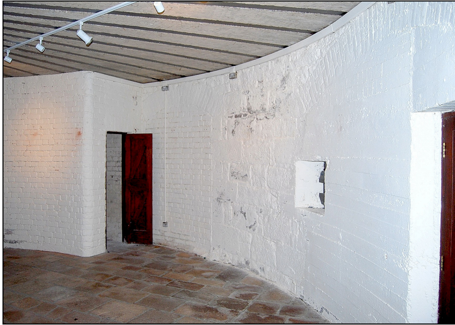
magazine showing blocked doorway (left) and German blocking (right)
