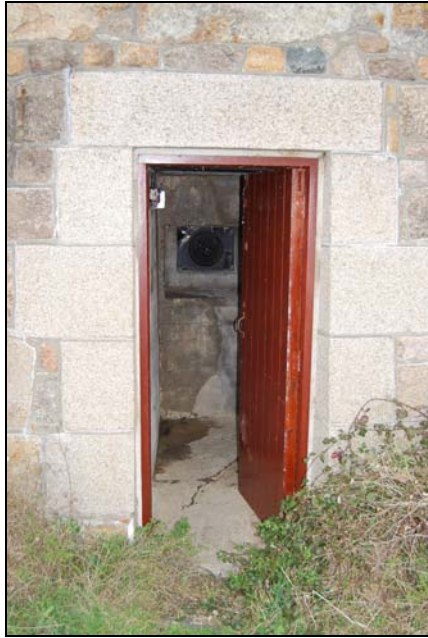
1941 entrance with machine gun position and steel blast door
