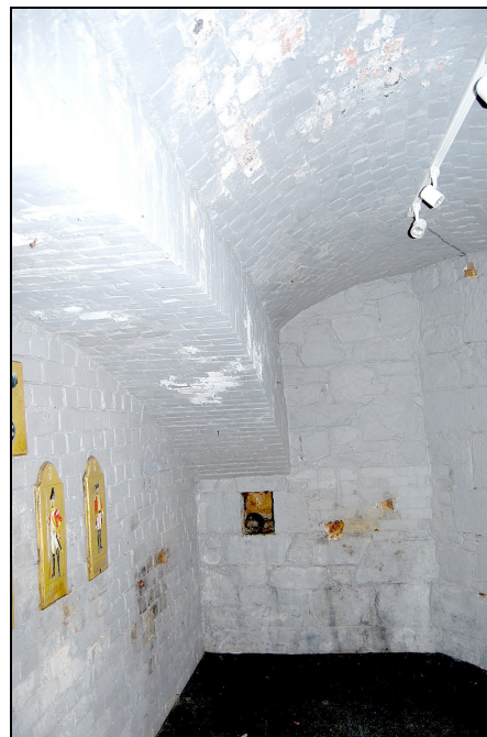
storeroom with baffled ventilation slot
