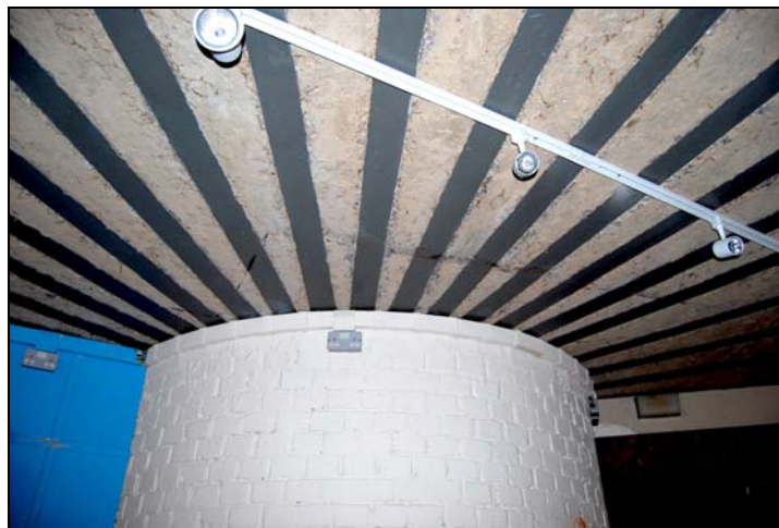
1941 radial steel and concrete floor
