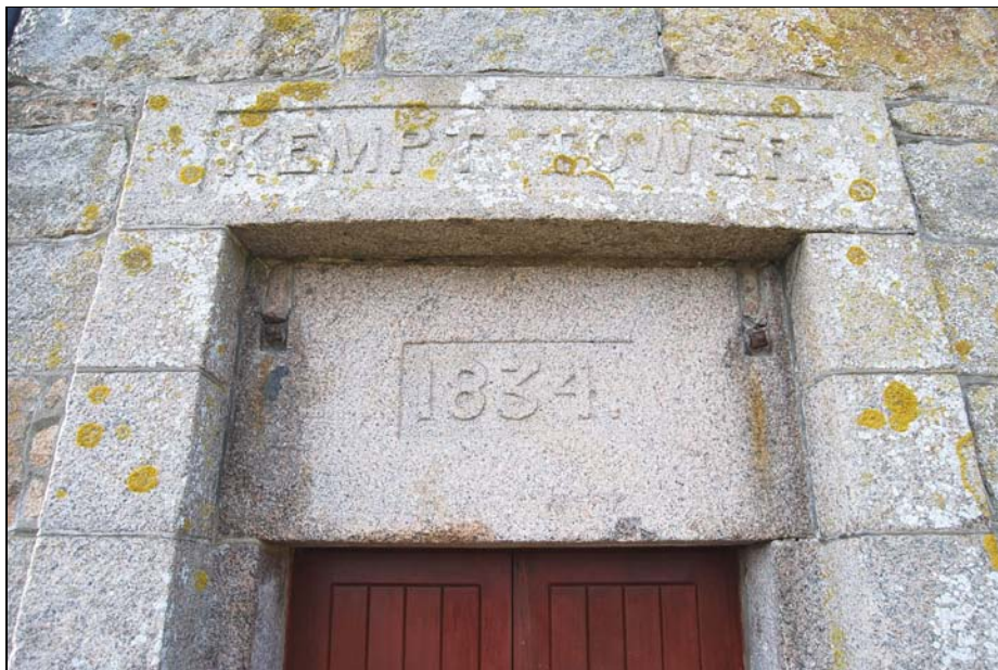
detail above original entrance
