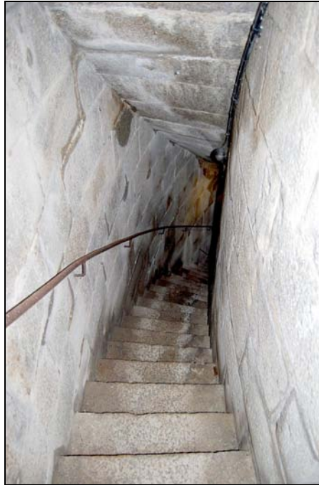
stairs within the thickness of external wall
