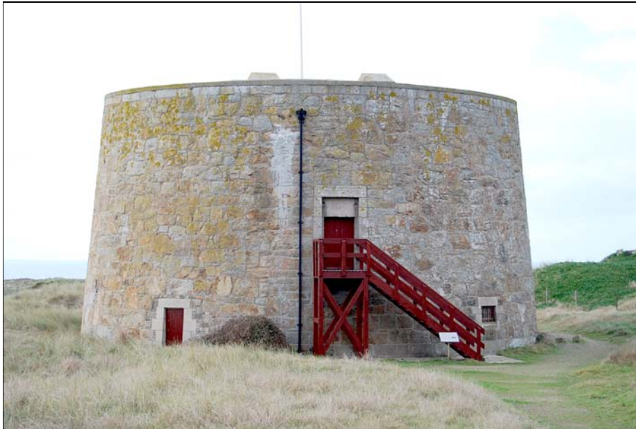
landward (west) elevation with original raised entrance flanked by 1941 insertions
