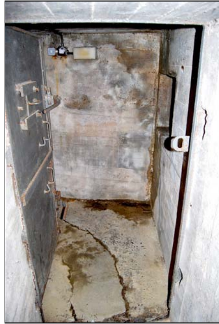
1941 entrance with machine gun position and steel blast door
