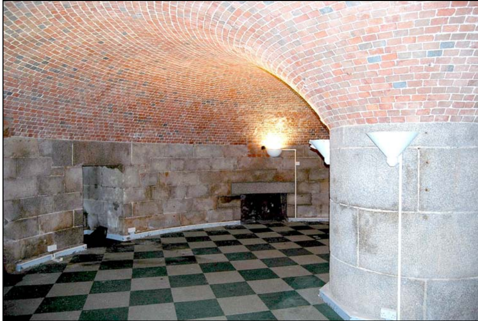
first floor accommodation level showing window and fireplace
