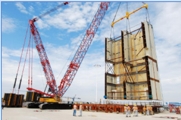
Haiyang – CA20 Subassembly 1 Moved into Integrated Assembly Platform
