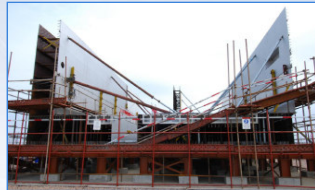
Haiyang – Assembly of CA20 Subassembly 3
