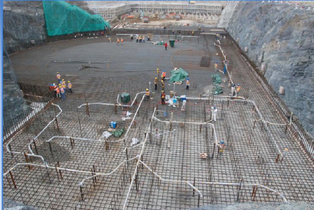
Sanmen - Bottom Mat and Drain Piping
