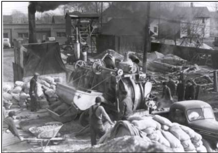
Figure 15 – Batching concrete aggregate using wheelbarrows and cement bags
