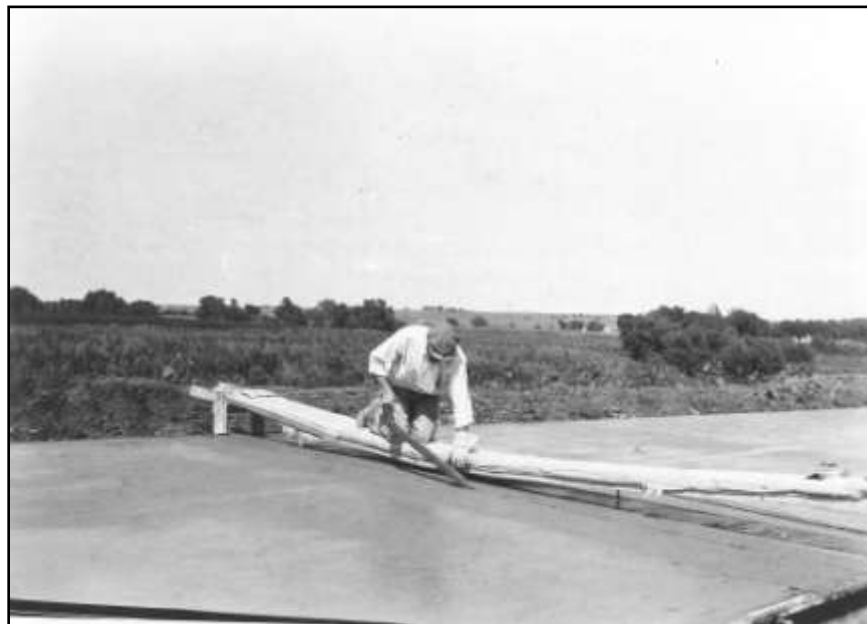
Figure 54 - Removing bituminous strip from expansion joint – Montgomery County 1930
