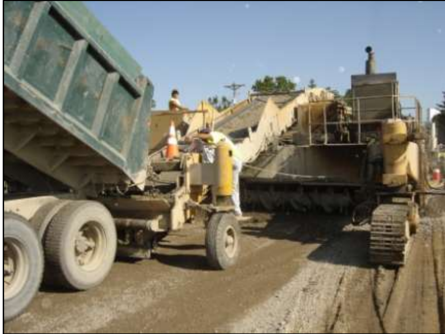
Figure 32 - Iowa Special trimmer/placer - Dallas County 2009
