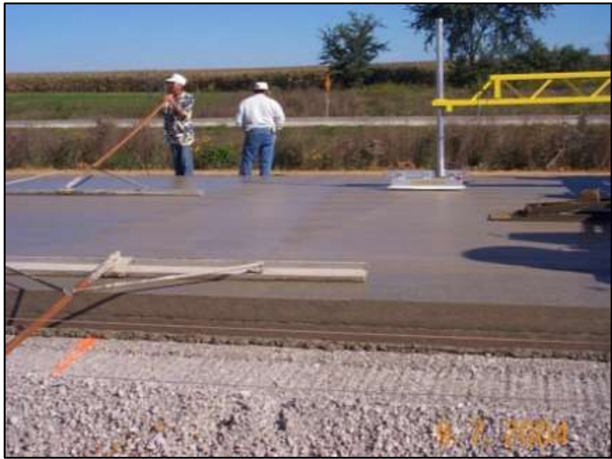
Figure 79 – Noncontact smoothness profile equipment (Ames Engineering)
