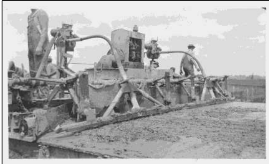
Figure 37 - Vibrators and tubes – Fayette County 1936
