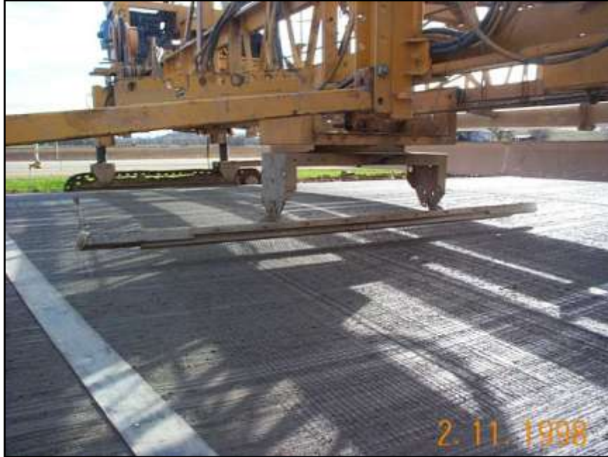
Figure 42 - Transverse tining - 1998
