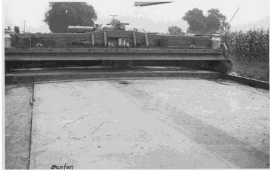
Figure 75 - PCC widening and resurfacing U.S. 30 Benton County 1949
