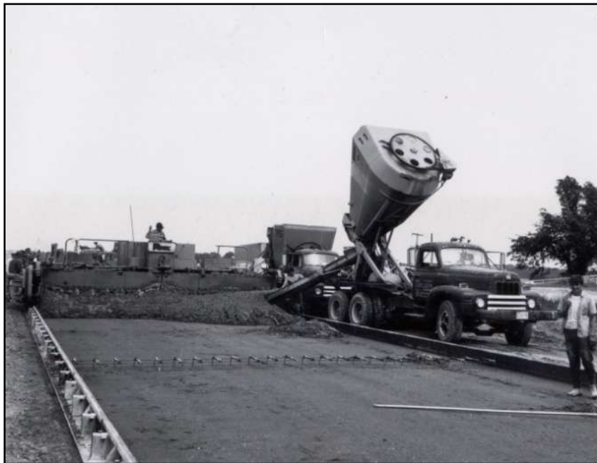
Figure 24 - Agitor truck dumping in front of paver – Dallas County I-80 1966
