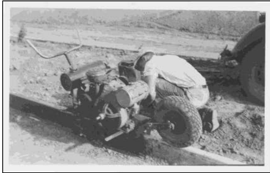
Figure 25 - Mechanical form tamper – Shelby County 1930s
