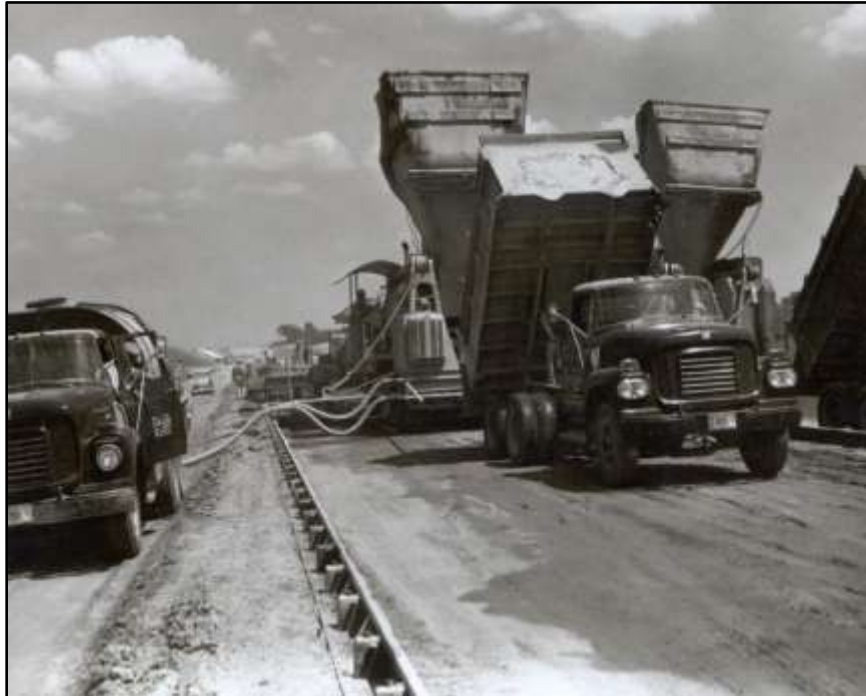
Figure 22 - Twin 34E mixers - Story County U.S. 30 1964
