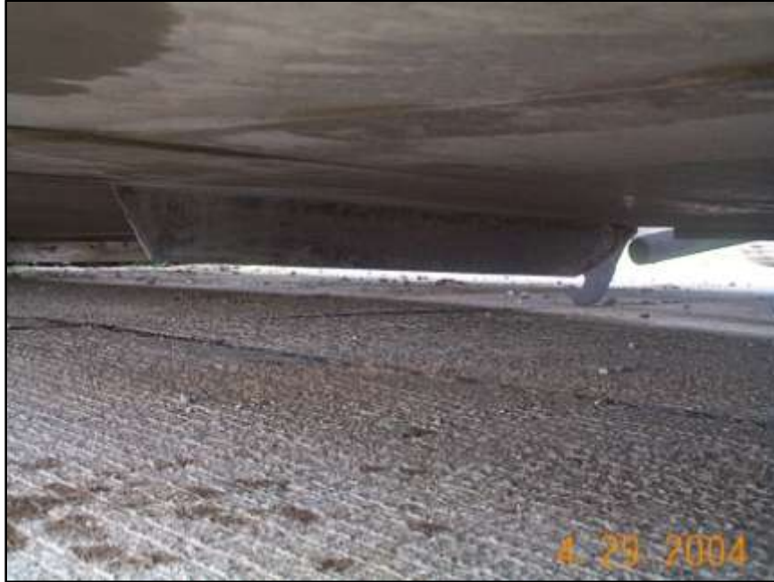
Figure 61 - Longitudinal joint forming knife on paver pan
