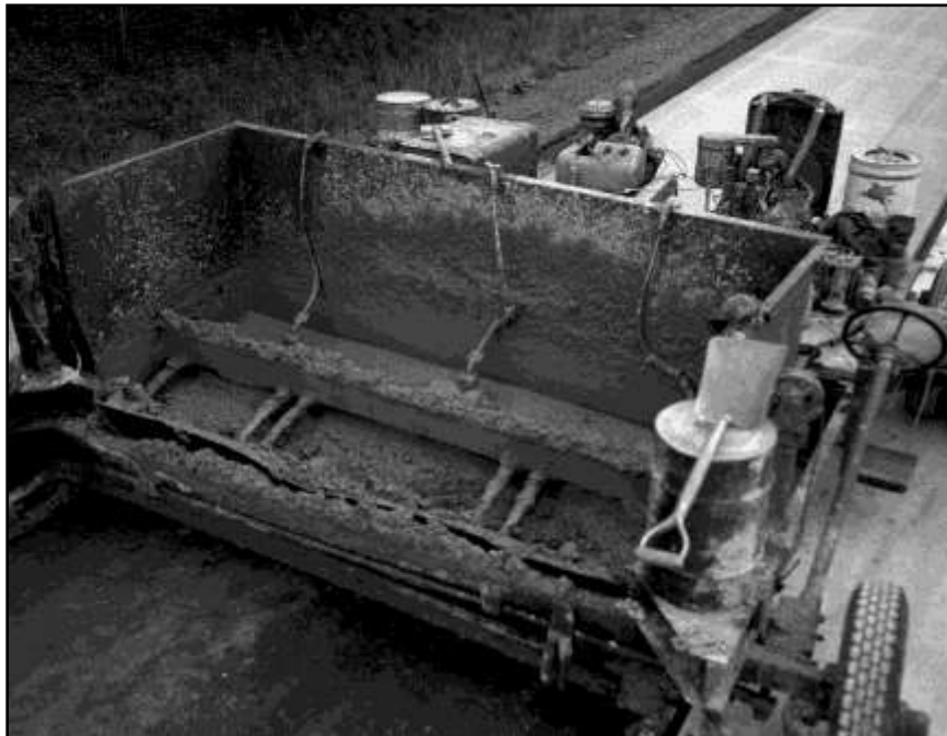
Figure 30 - Johnson slip form paver closeup - 1954
