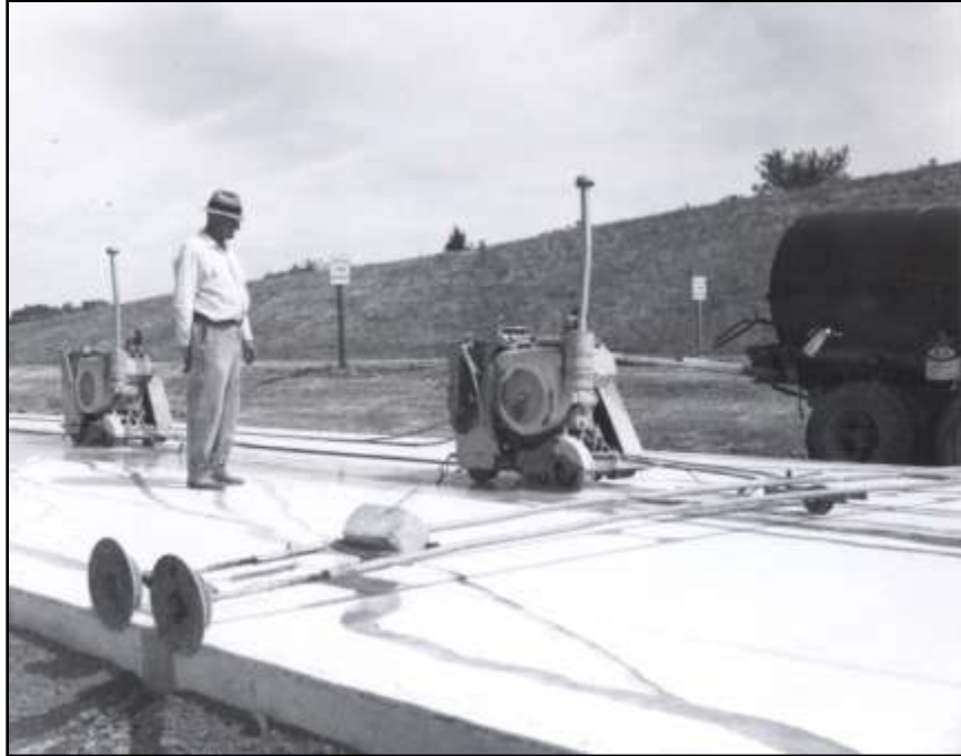
Figure 59 - Sawing longitudinal joint – Dallas County 1966
