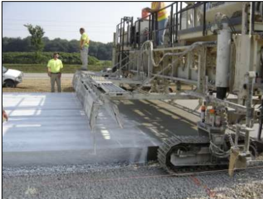
Figure 49 - White pigmented curing - Tama County 2005
