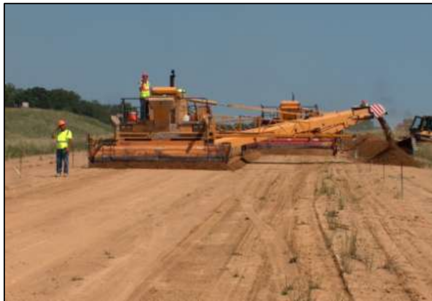
Figure 4 – Modern subgrade trimmer
