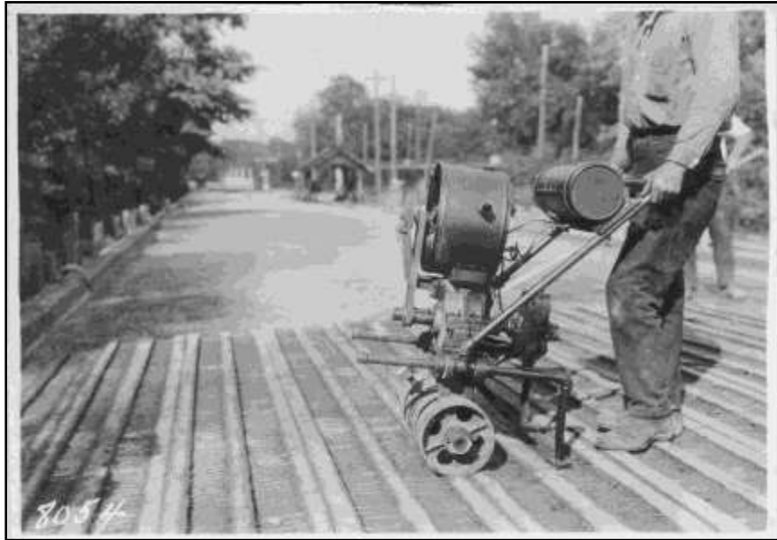
Figure 28 - Mechanical tamping and boards – Blackhawk County 1921
