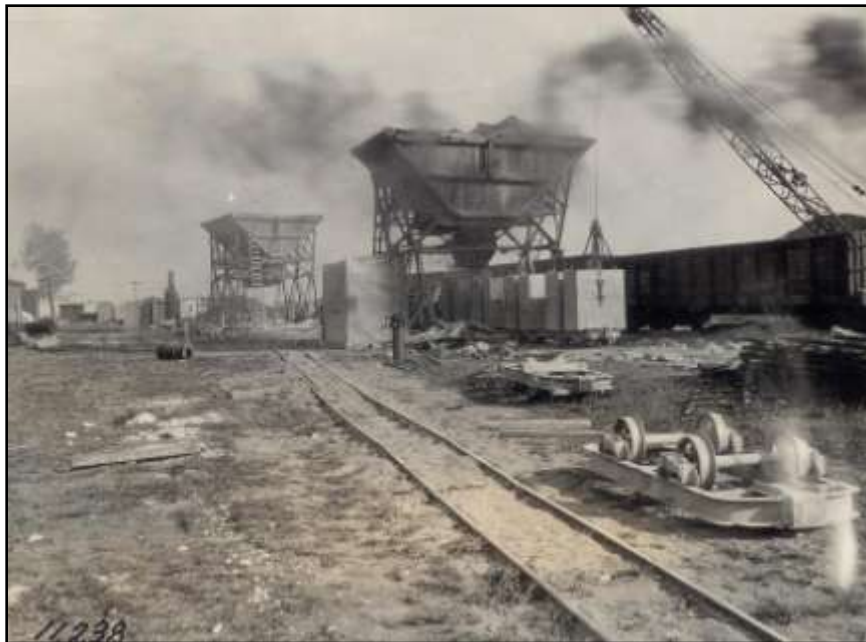
Figure 19 - Aggregate batch plant and rail lines – Wapello County 1926
