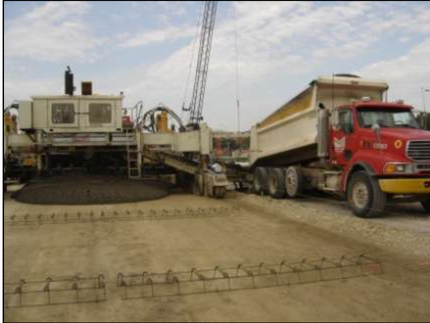
Figure 33 - Dump truck and belt placer/spreader - Polk County 2006
