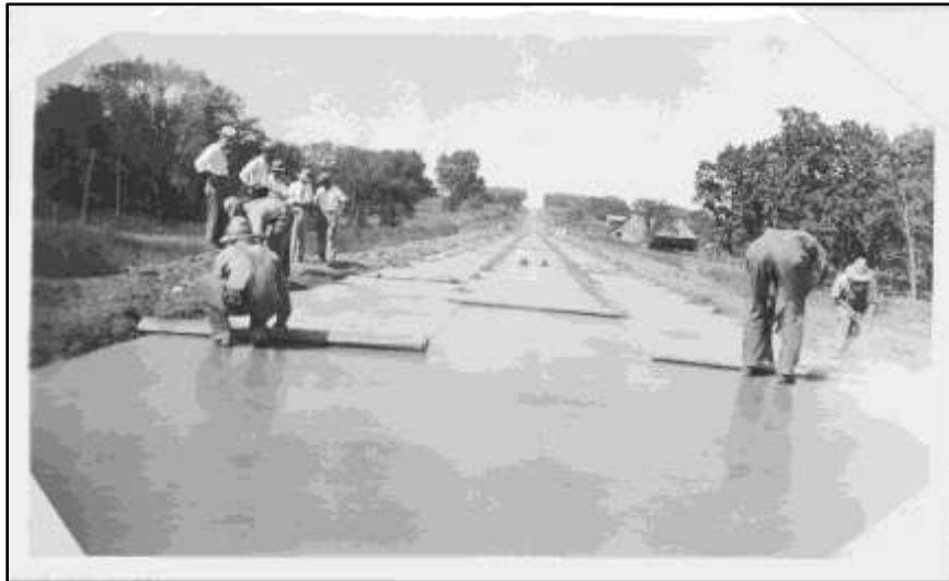
Figure 47 – Sisalkraft paper curing – Washington County 1930
