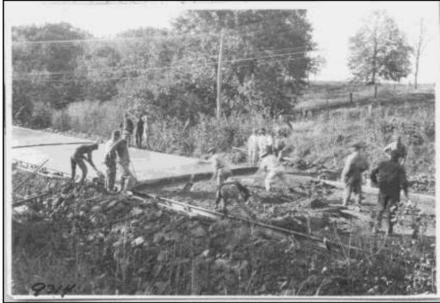
Figure 26 - Striking off concrete by hand – Story County 1922
