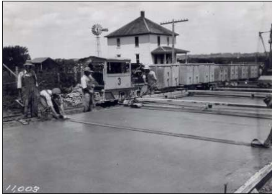
Figure 41 - Belting surface – Polk County 1926
