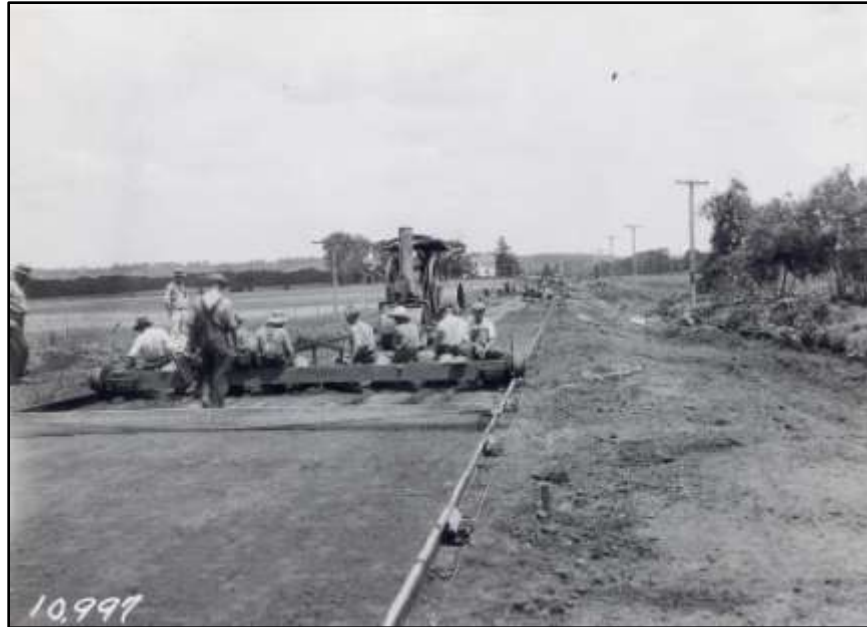
Figure 3 – Subgrade trimmer and template – Polk County 1926
