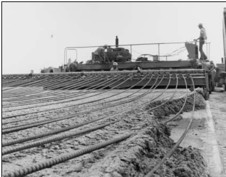
Figure 73 - CRC steel fed through machine - Franklin County I-35 1976
