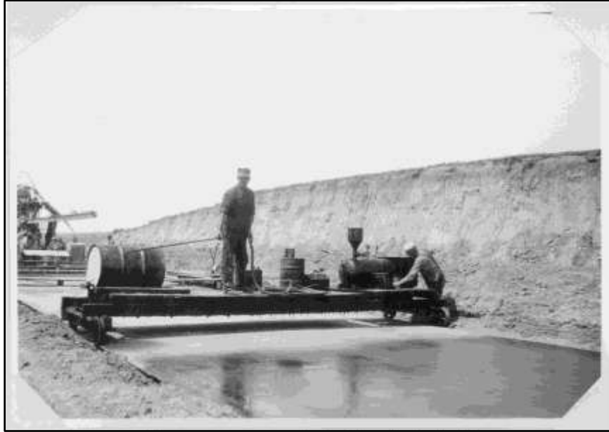
Figure 48 – Curecrete bituminous curing - Pottwattamie County 1920s
