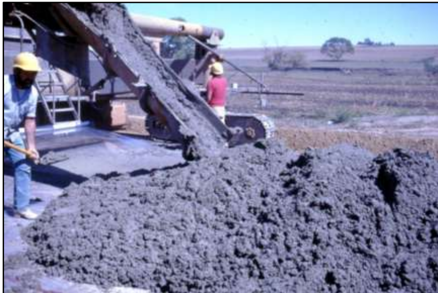
Figure 6 - Plastic sheet placed on subgrade behind Iowa Special paver – Lyon County 1977
