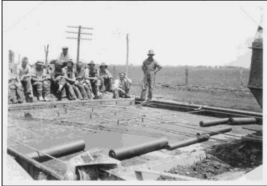
Figure 5 - Placing tar paper on subgrade - Story County 1926
