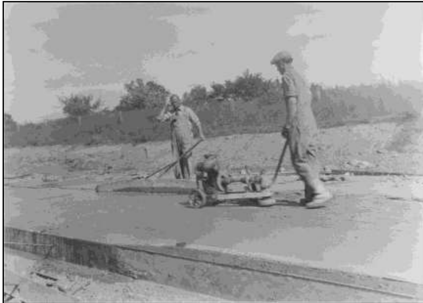
Figure 63 - Surface correction with carborundum brick – Keokuk County 1932
