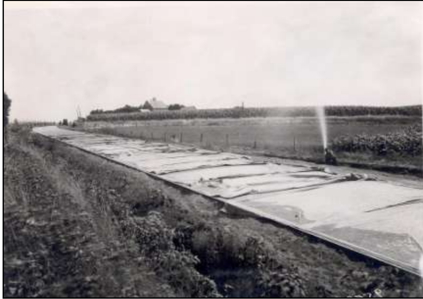
Figure 44 - Burlap and water curing – Woodbury County 1921
