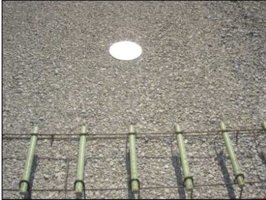
Figure 80 – Metal target before placement to test pavement thickness
