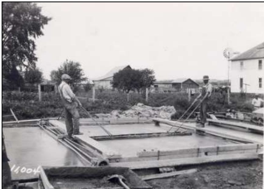
Figure 40 - Longitudinal finishing – Polk County 1926
