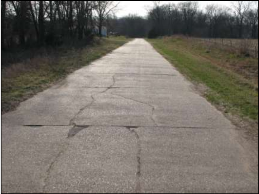
Figure 51 – Moscow Road Muscatine County 1914 - formed transverse joints at 25 foot intervals
