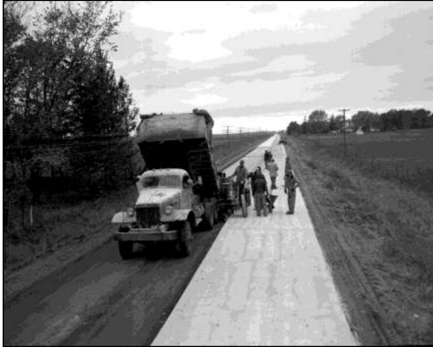
Figure 29 - Johnson slip form paver Greene County 1954
