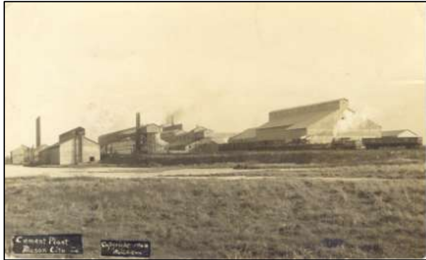
Figure 13– Northwestern States cement plant 1908- from the collection of Hank Zaletel.
