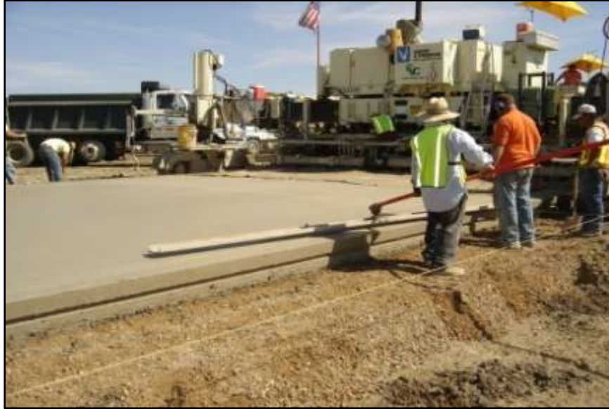
Figure 35 - Guntert-Zimmerman slip form paver - Osceola County 2007
