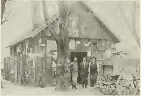
Outside of the John Bolden Blacksmith Shop
