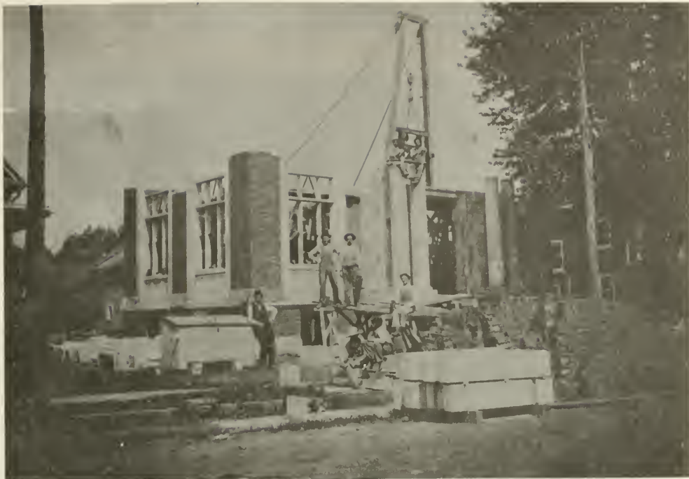
DURING THE CONSTRUCTION OF THE LIBRARY
