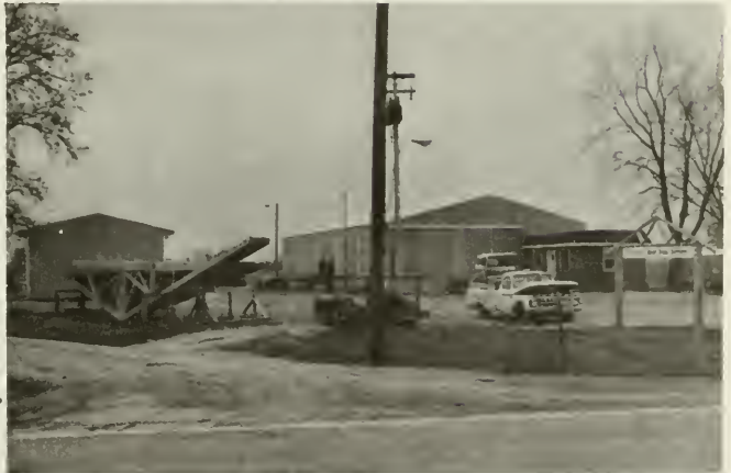
Component Roof Truss System factory, north of railroad on Rt. 1
