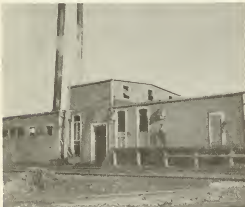
The Ice Plant at Ridge Farm
