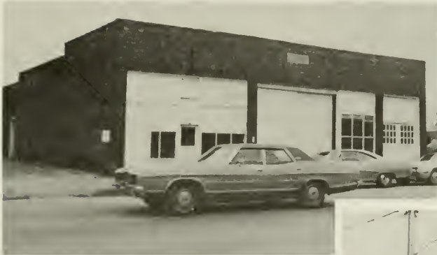
East Side of South State Street. Left side of the building was the Inter-urban Station
