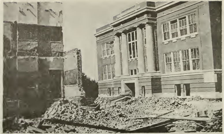
The new school standing over the rubble of the old 1911
