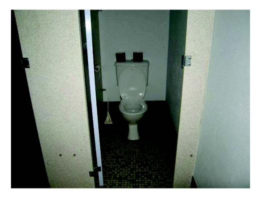
**Figure 12** Photograph of interior of office building – Toilets do not have dual flush cisterns and the floor and wall tiles require replacing.
