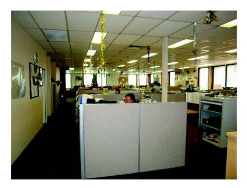
**Figure 10** Photograph of 4.002, (same condition as 4.003, 4.005 and 4.006) - Ceiling grid and tiles require replacement due to their condition and the water marks.
