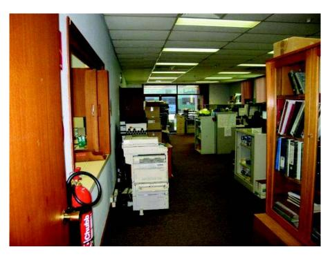
**Figure 7** Photograph 1.001, (same condition as 1.002, 1.003, 1.004 and 1.011) Ceiling grid and tiles require replacement due to their condition and the water marks.
