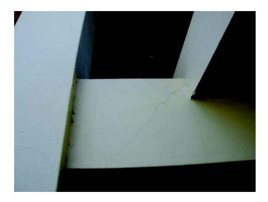
**Figure 13** Exterior of office building – Cracking less than 1mm was evident on external walls, beams, columns and edges of concrete slabs.
