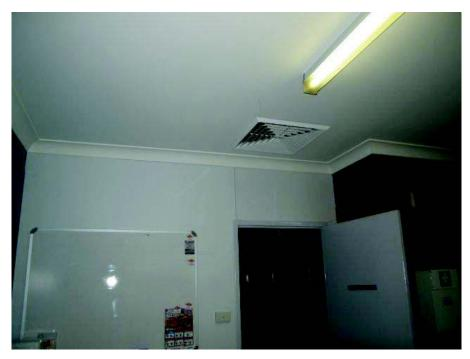
**Figure 8** Photograph of 2.001 (same condition as 2.005 and 2.008) – Ceiling grid and tiles require replacement due to their condition and the water marks.
