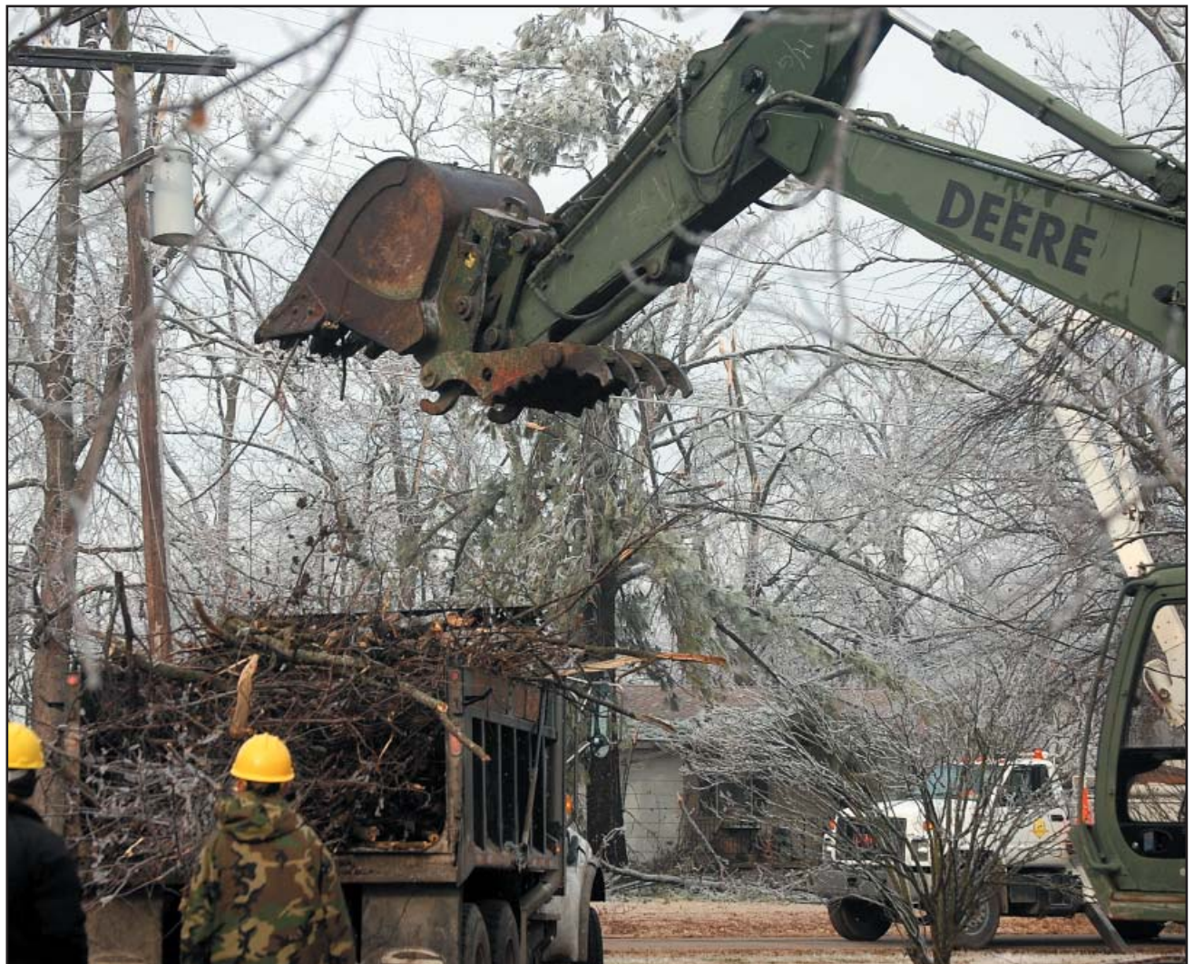
lines and choked public roads. The debris that blocked public thoroughfares was scooped, lifted, sawn and dumped into waiting trucks to be hauled away. (Photos by Sgt. Steve Perkins)
