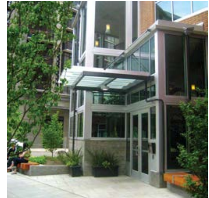
Good Example of Visible and Weather Protected Entrance, Site Furnishings, and Transition from the Street
