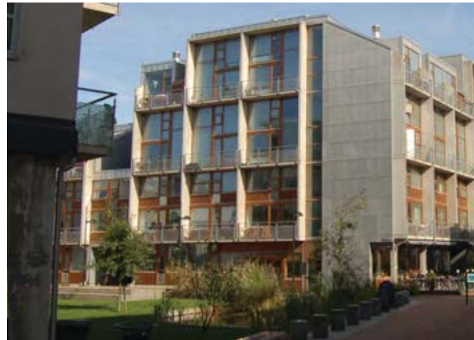
Building stepping down and back
