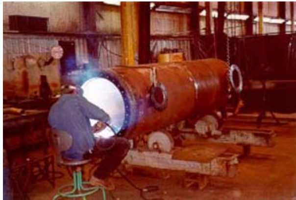
Welding the shell
