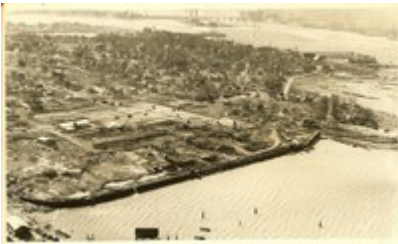
Construction of the Todd-Bath Yard in early 1941, this yard was later referred to as the East Yard.
