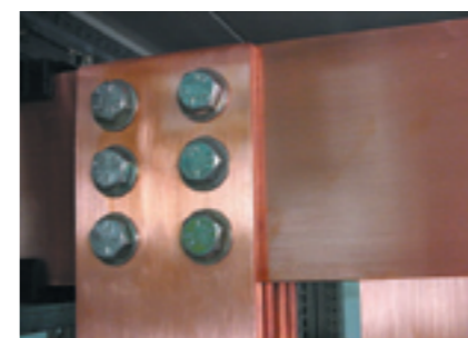
^ Connection on 120 x 10 bars (4000 A)
