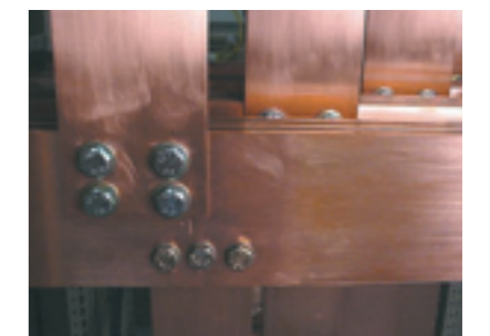
^ Double connection: 100 x 10 bars (3200 A) and 80 x 10 bars (2500 A) on common 120 x 10 bars
