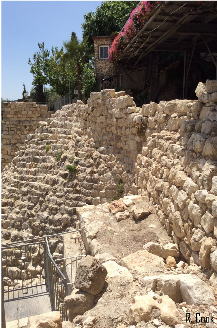
City of David Stepped stone retaining wall
