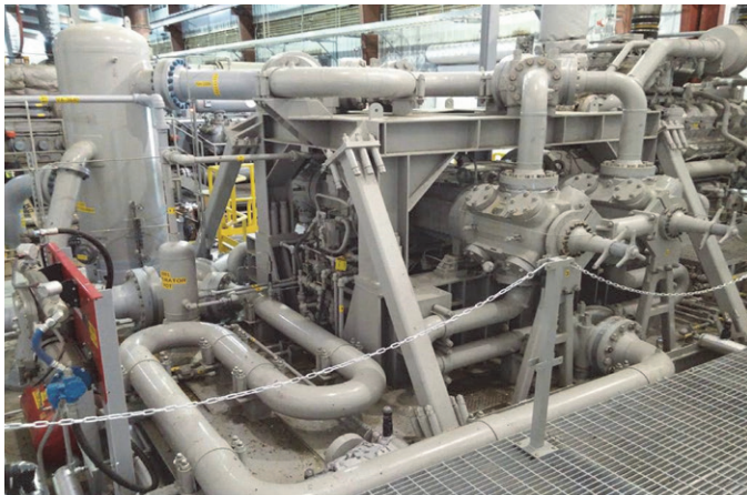
Figure 11: Second PAN Manifold unit installed (with work platforms) – left side view.
