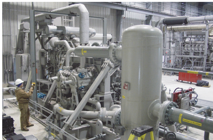
Figure 7: First PAN Manifold unit installed (without work platforms) – left side view.
