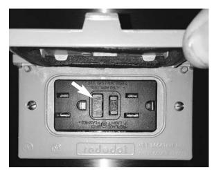
Figure 4-2. Reset Button on GFCI Outlet
