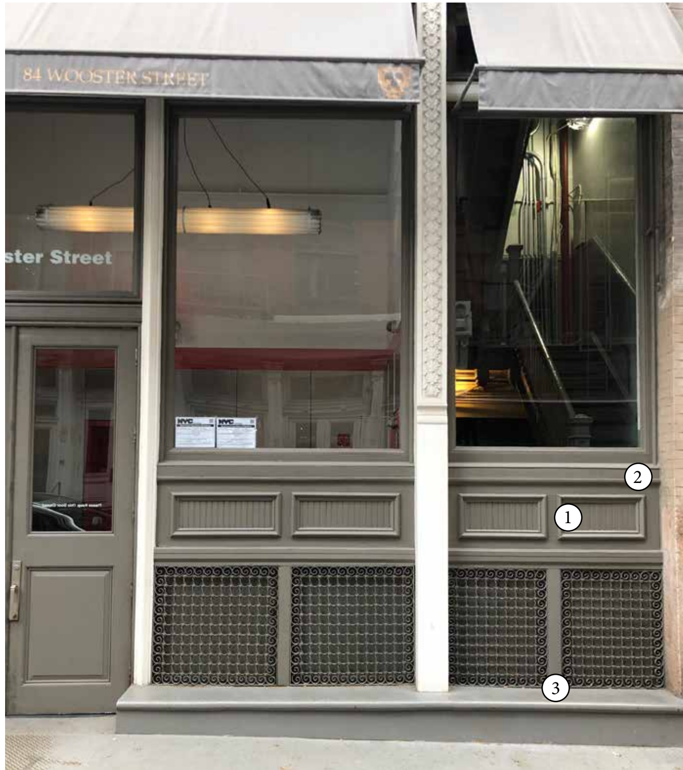
84 WOOSTER STREET WINDOW BAY
