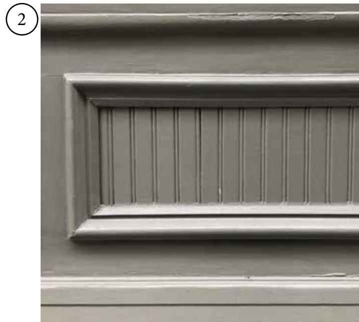
EXISTING WOOD/PLYWOOD BULKHEAD PANEL (NOT HISTORICAL. TO BE REMOVED)
