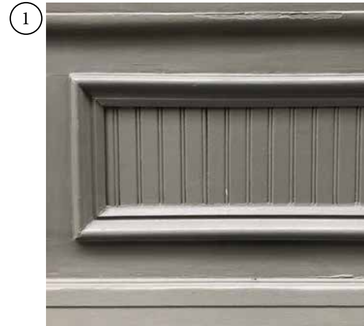
EXISTING WOOD BULKHEAD PANEL (TO BE REMOVED)
