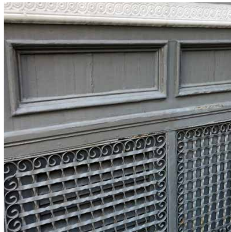
WALL MATERIAL DETAIL PHOTO
