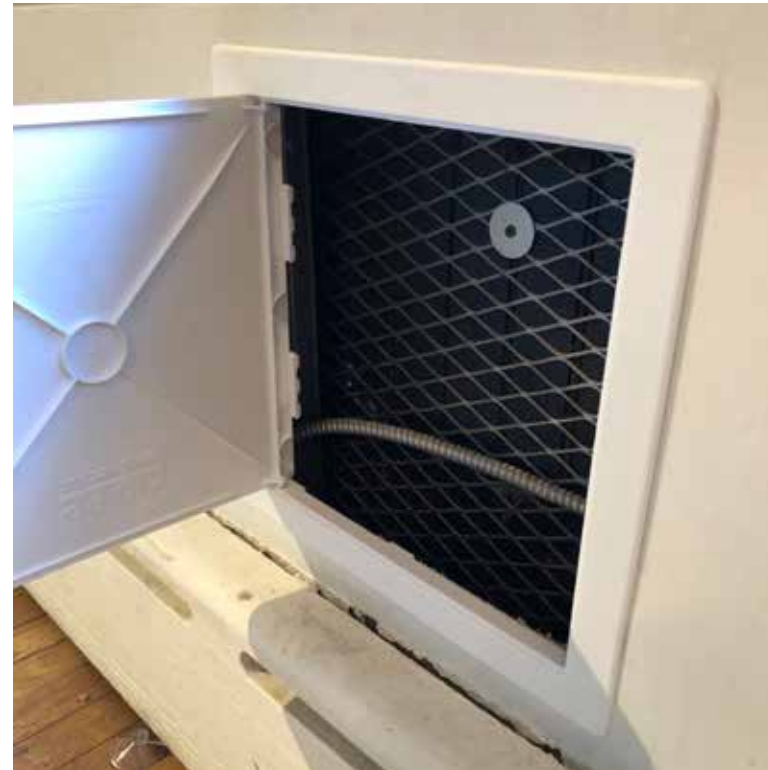
WALL ASSEMBLY DETAIL PHOTO
