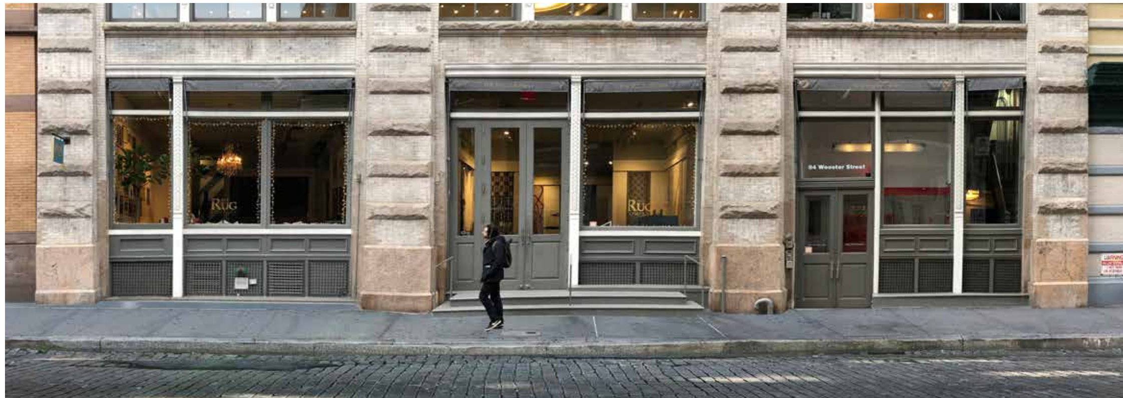
84 WOOSTER STREET - EXISTING STOREFRONT
