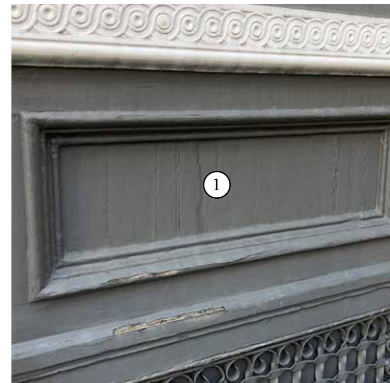
WALL MATERIAL DETAIL PHOTO
