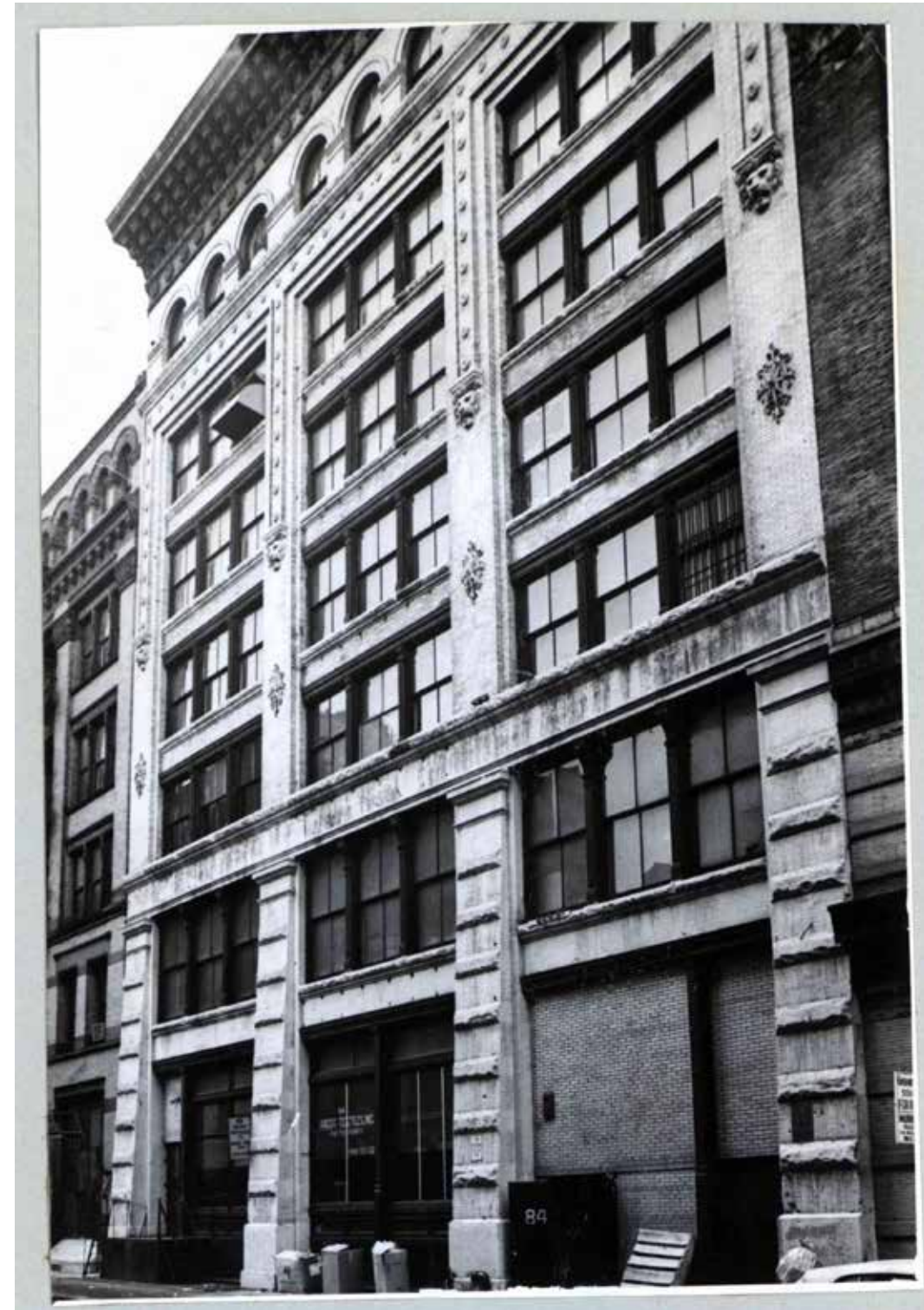
84 WOOSTER STREET - 1970'S LPC DESIGNATION PHOTO
