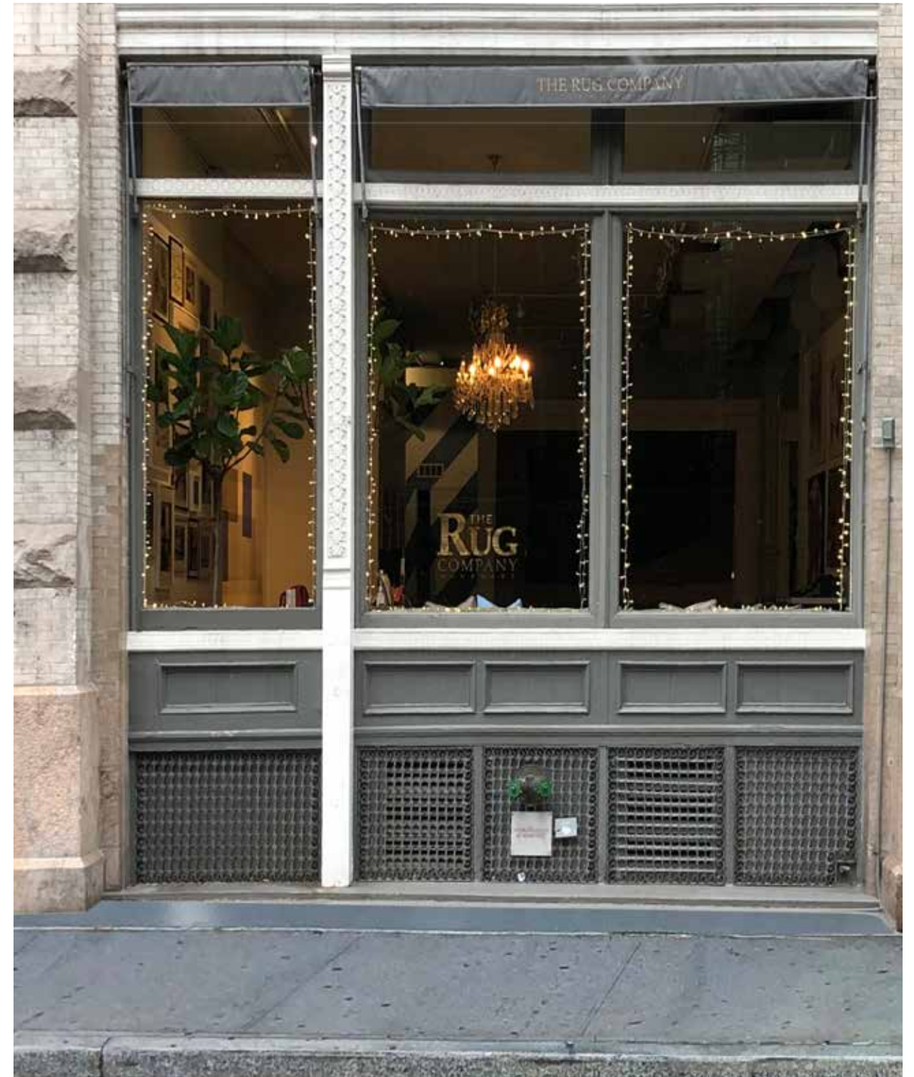
84 WOOSTER STREET DUAL PANEL BULKHEAD
