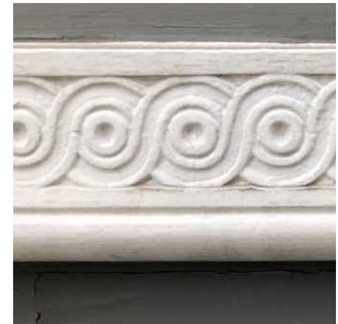
TYPICAL EXISTING HORIZONTAL CAST IRON DETAIL
