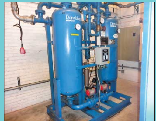
Air Cel Model AHLD-750 Desiccant Air Dryer
