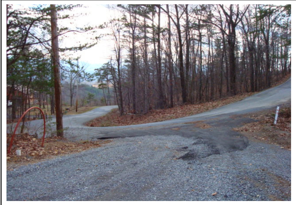
Bluff Mountain Road from Entrance
