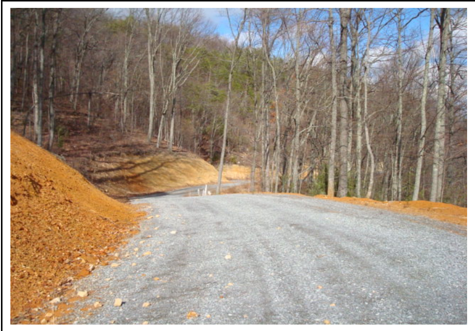
Viewing East on New Access Road
