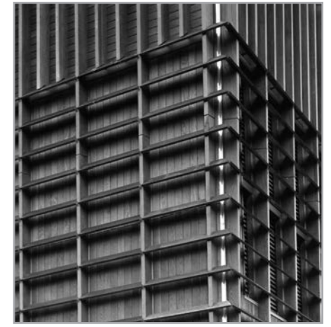
Detail of cladding to external corner to service building. The timber louvres are used as a scaling device and to hide the aluminium louvres behind.
