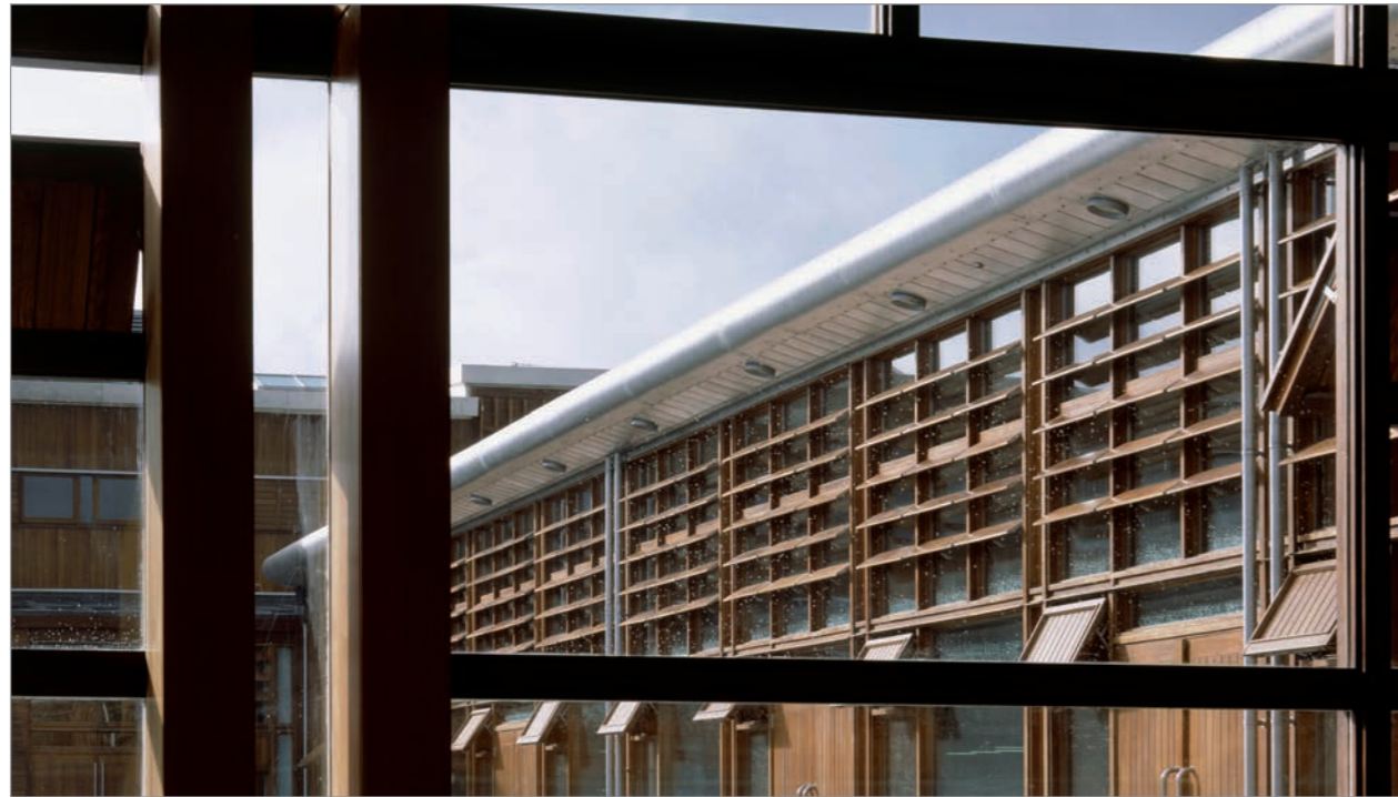
European Commission Food and Veterinary Office, Grange, Co.Meath. View of internal courtyard and timber screen with integrated louvres.
