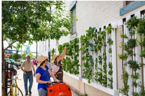
(installation by Bright Agrotech, Laramie, USA)
