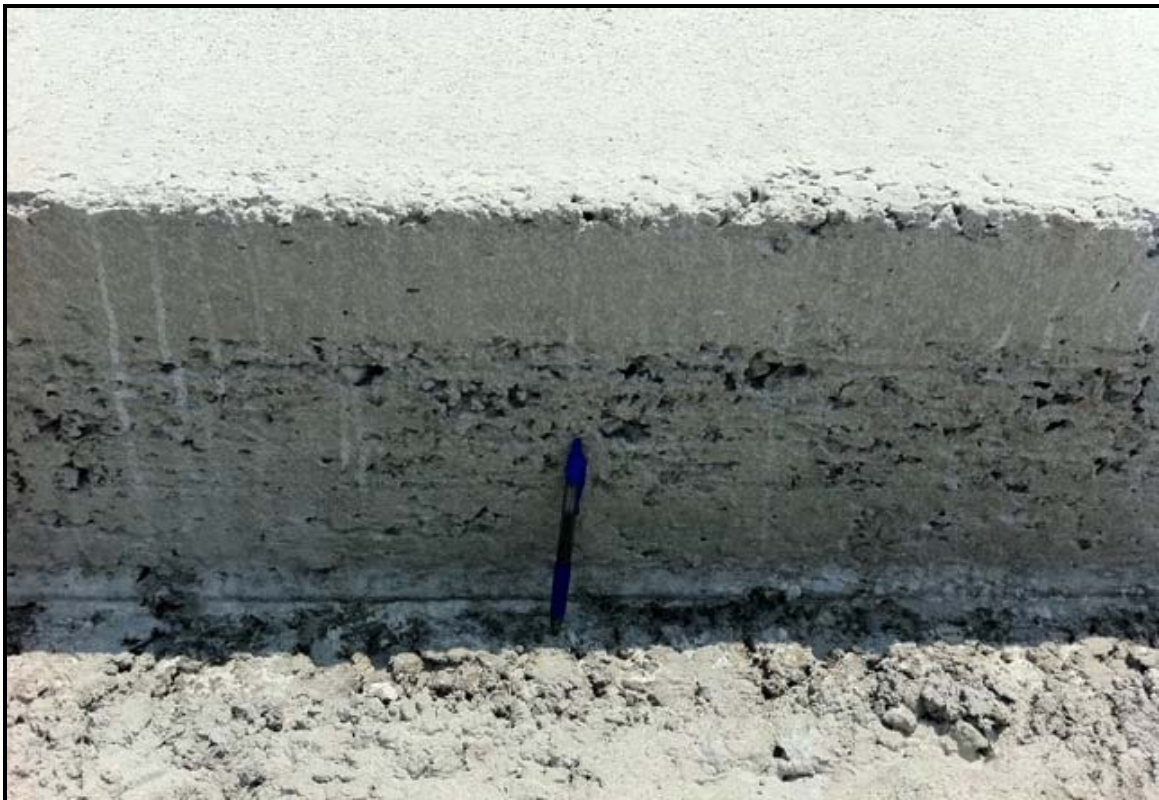
Figure 16. Rough Edge and Side Face of Slipform HTC
