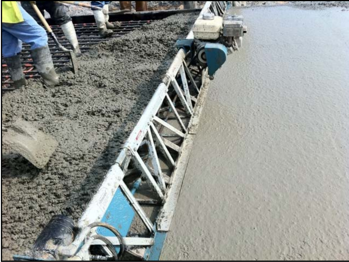
Figure 14. Vibrating Truss Screed
