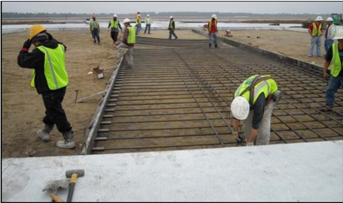
Figure 7. Placing Continuous Reinforcement
