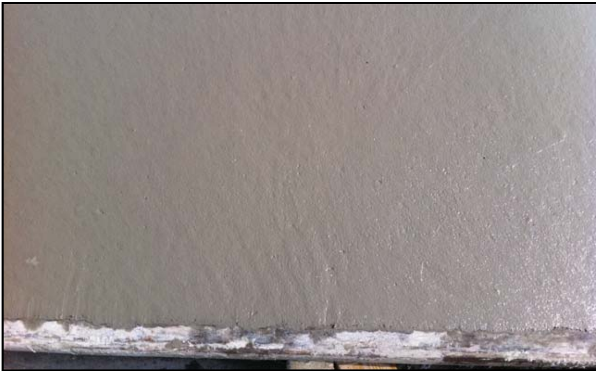
Figure 19. Final HTC Surface Prior to Brooming
