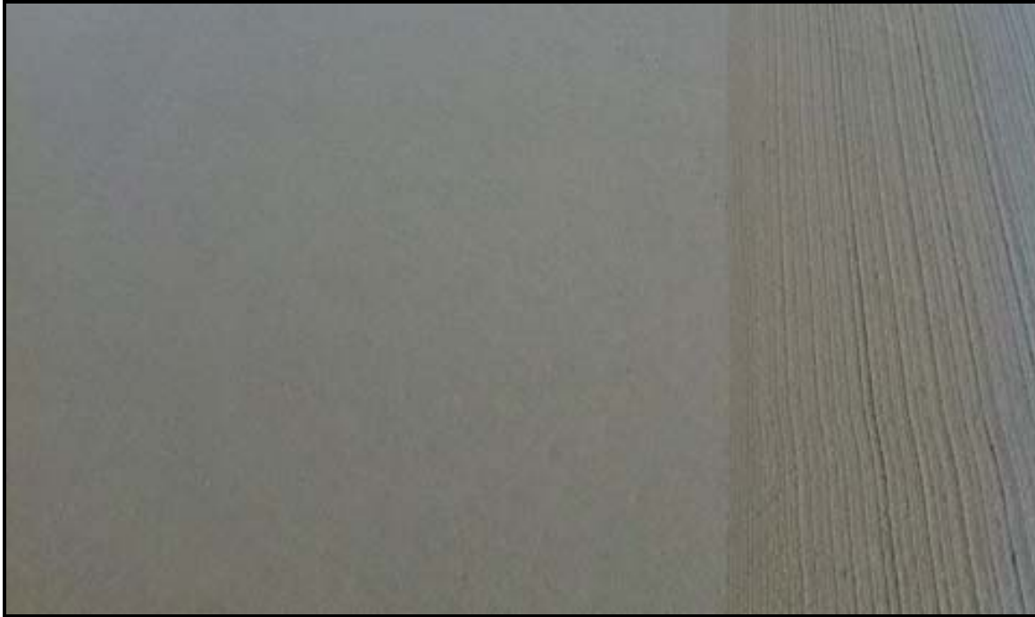
Figure 22. Unbroomed and Acceptable Broomed Surfaces
