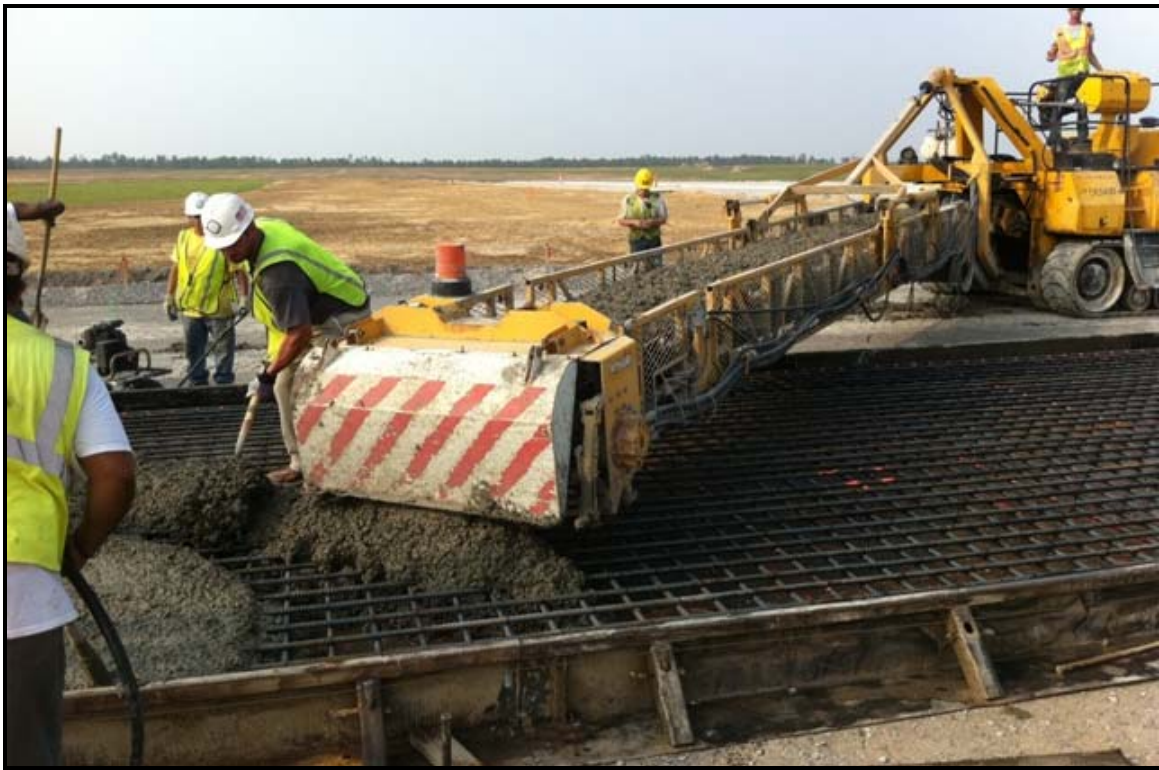
Figure 13. Conventional Belt Placer - Not Allowed
