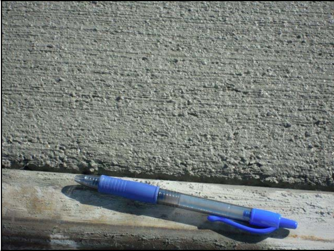
Figure 21. Unacceptable Broomed Surface
