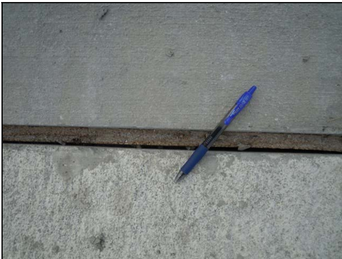
Figure 23. HTC Shrinkage at Isolation Joint
