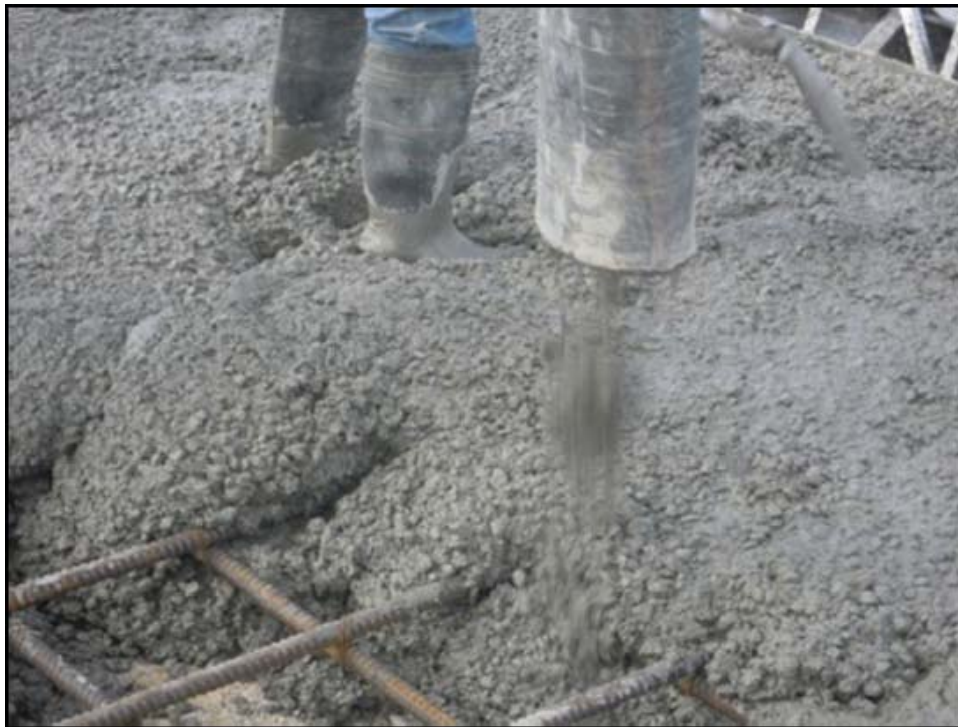
Figure 11. Conveyor Discharge
