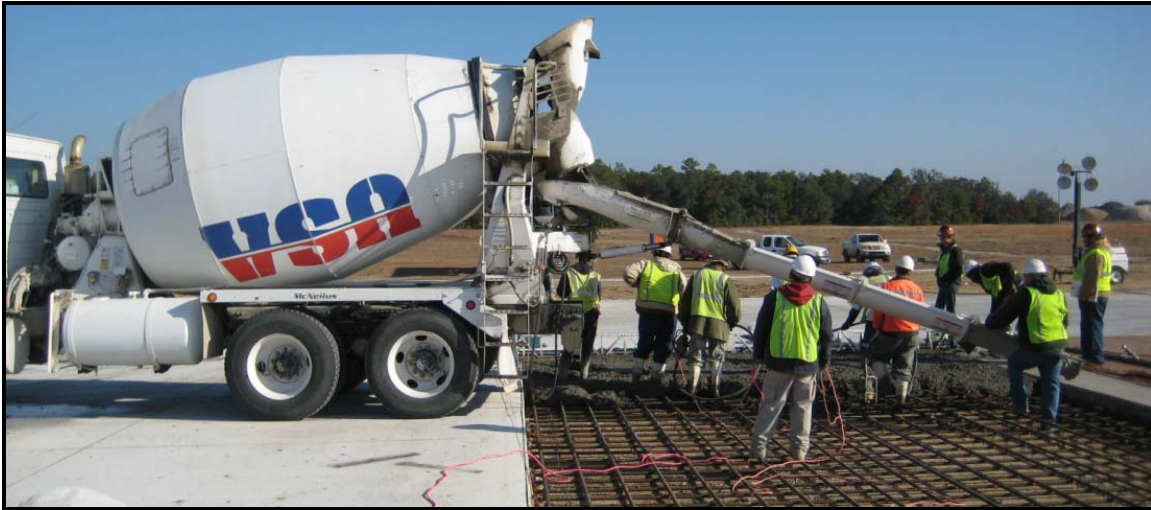
Figure 12. Direct Discharge from Ready-Mix Truck
