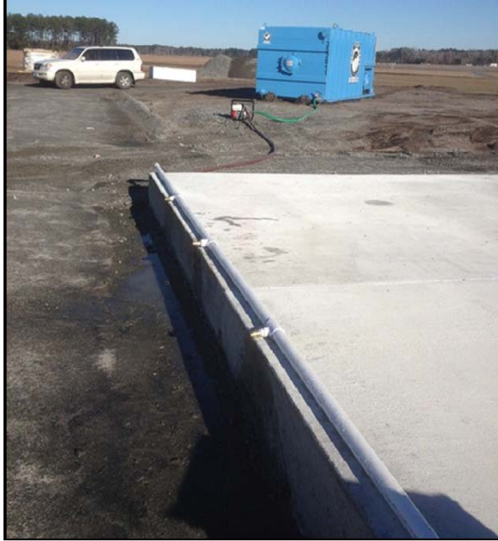
Figure 24. Auxiliary Water Tanks and Manifold, MCAS Beaufort
