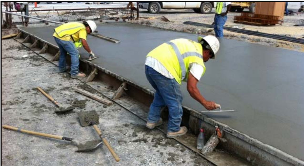
Figure 18. Final Finishing with Channel Float and Hand Tools
