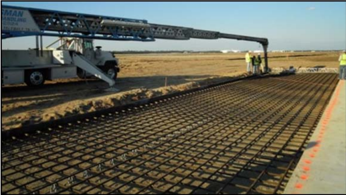
Figure 10. Telescoping Conveyor
