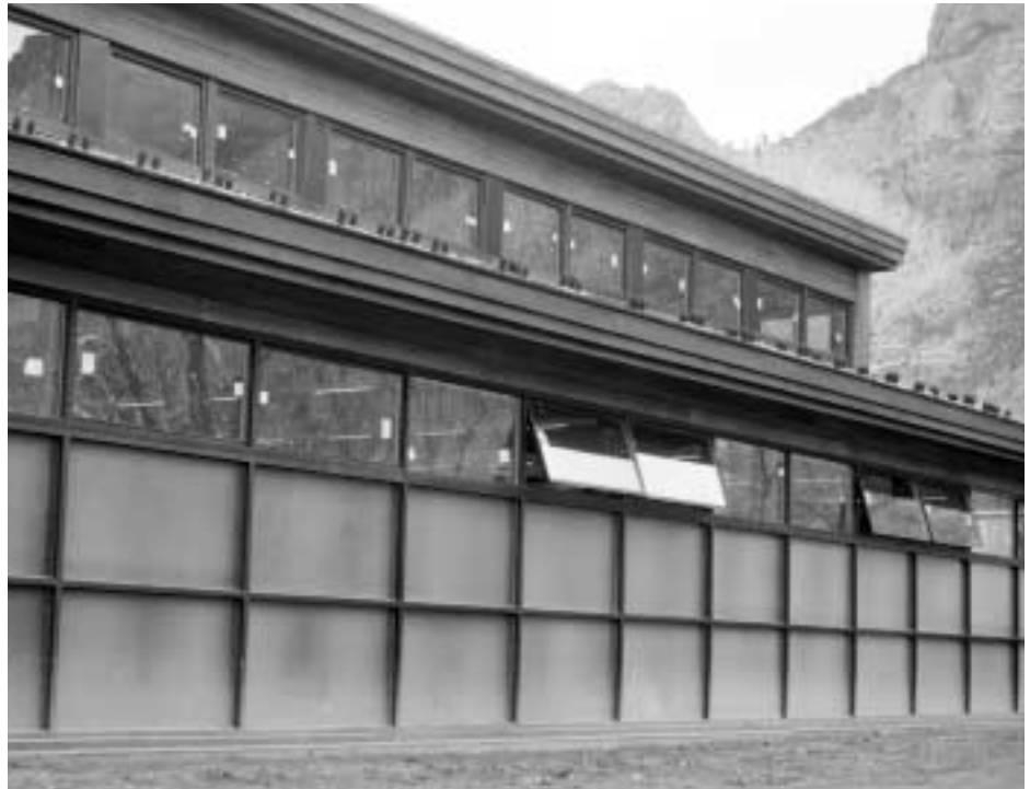
The Trombe wall provides most of the heating for Zion National Park Visitor Center. Heat from the sun is trapped between a pane of glass and a black selective coating. A masonry wall stores the heat for release into the building later in the day.
