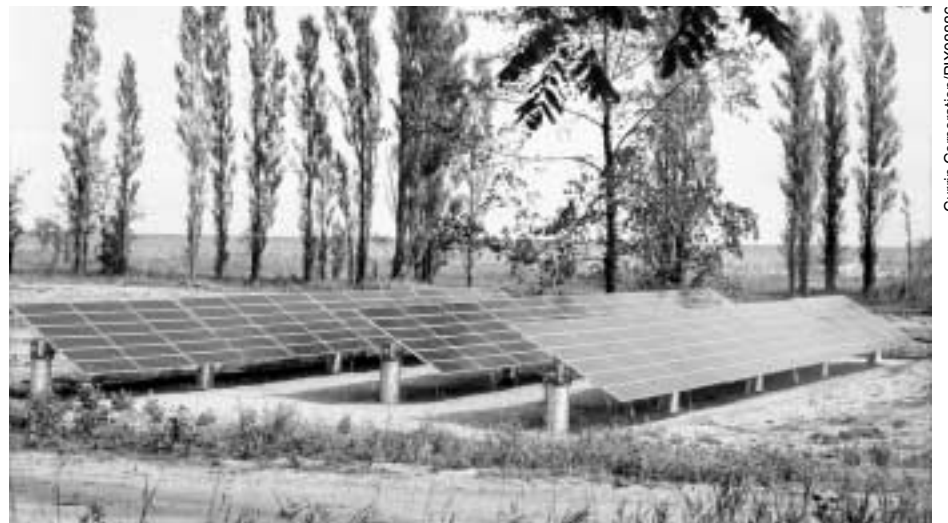
A new 10-kW hybrid PV/diesel generator system protects the wilderness area on North Manitou Island by significantly reducing the noise and air pollution caused by the old diesel generator system.
