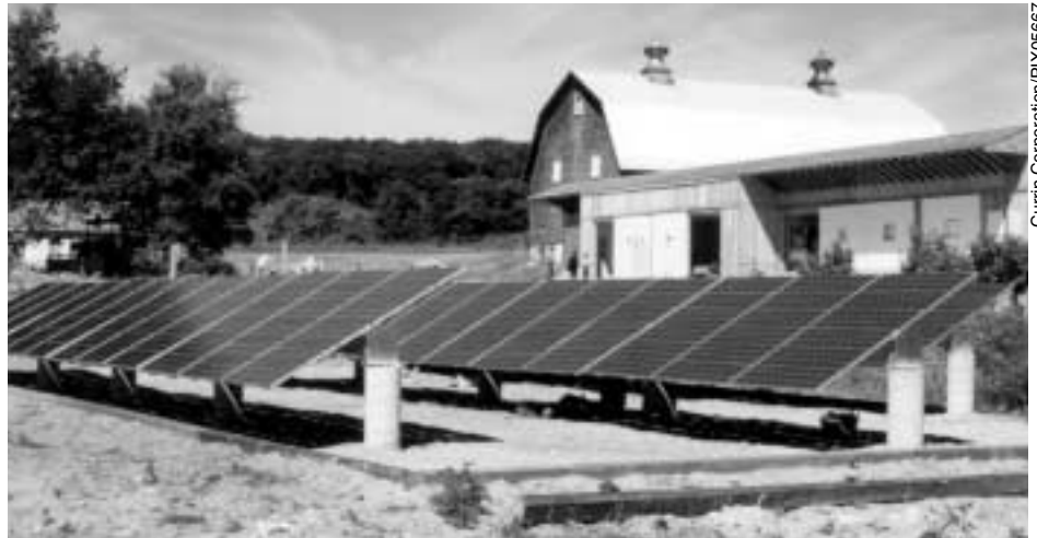
A hybrid PV/diesel generator system provides energy to the historically significant buildings that house administrative offices on North Manitou Island in Sleeping Bear Dunes National Lakeshore, Michigan.
