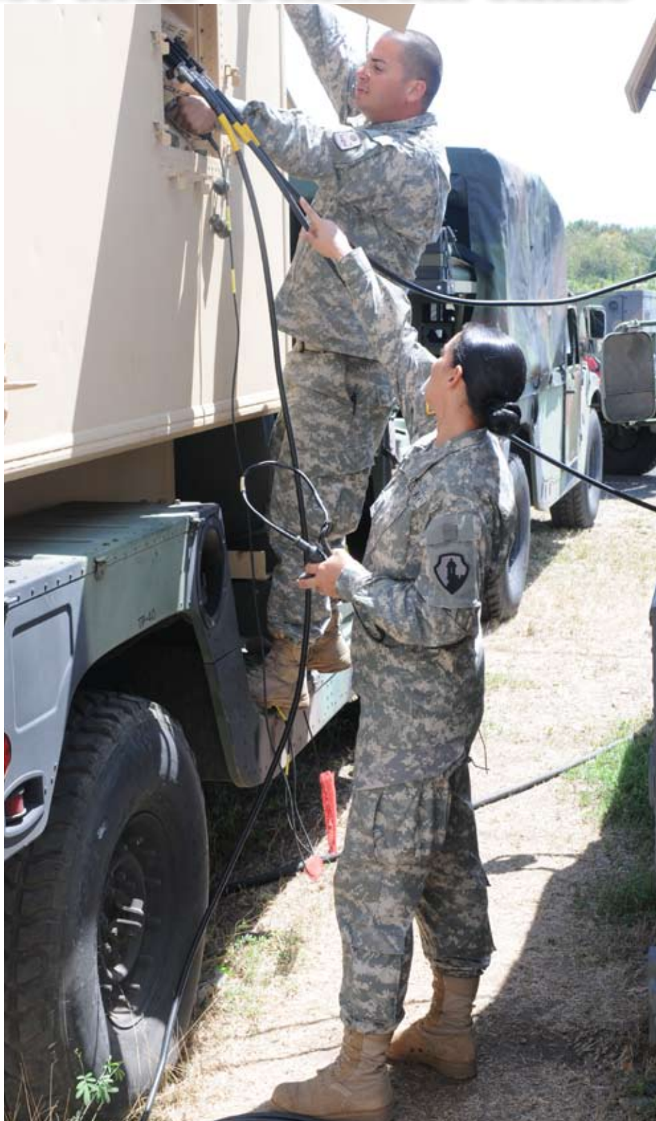
Soldiers troubleshoot a connection by replacing a coaxial cable in one of the communication shelters, at Camp Santiago Joint Maneuver Training Center, earlier during the year.
