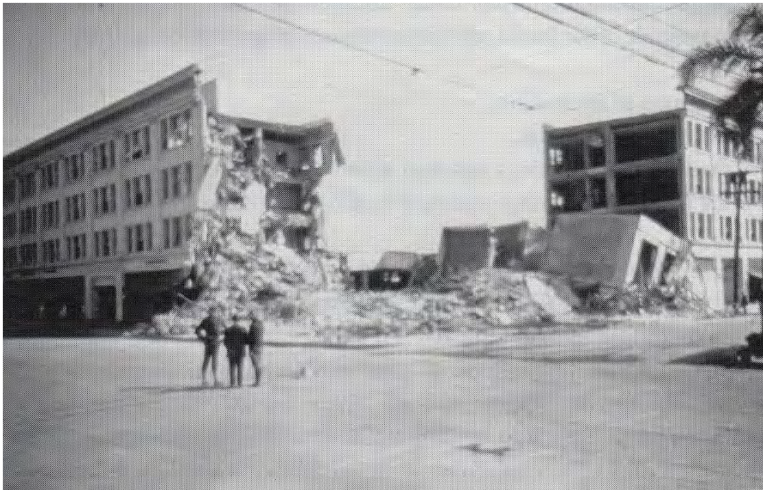
Collapse of the L-shaped San Marco Building in the 1925 Santa Barbara California earthquake.
