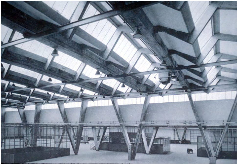
Maintenance building at Fiumicino Airport, Rome Italy. Ricardo Morandi ca. 1960
