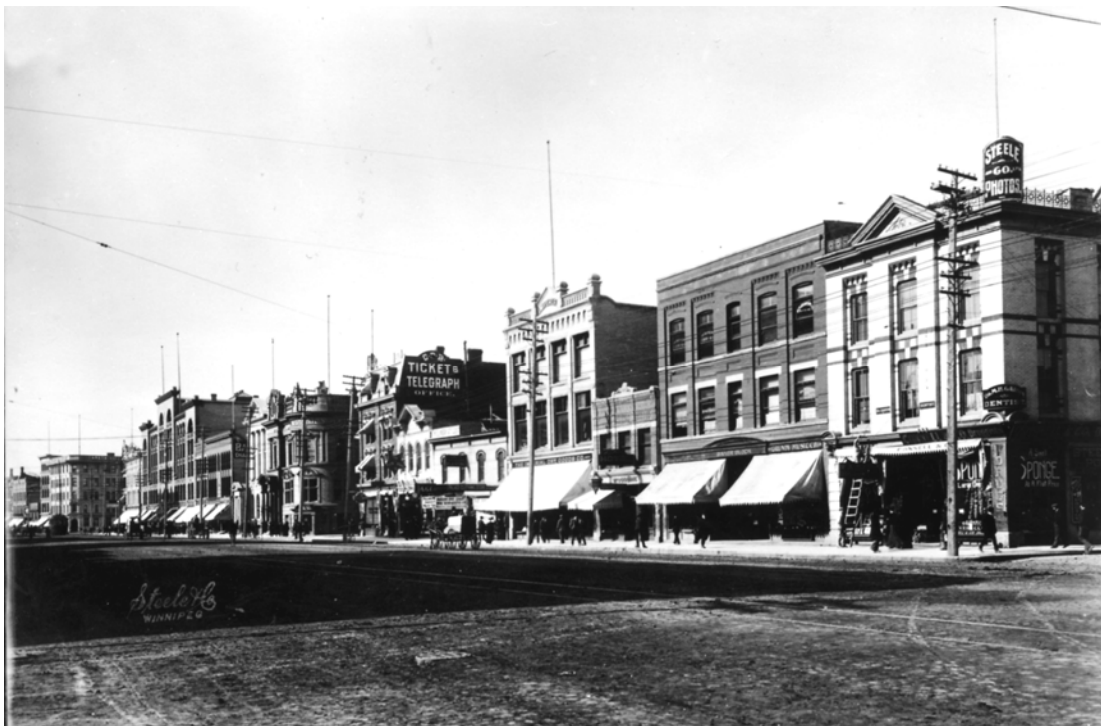
View of Main Street in Winnipeg, c. 1915 (Archives of Manitoba). Even a small collection of buildings of broadly similar architectural character contains a wealth of different styles.
