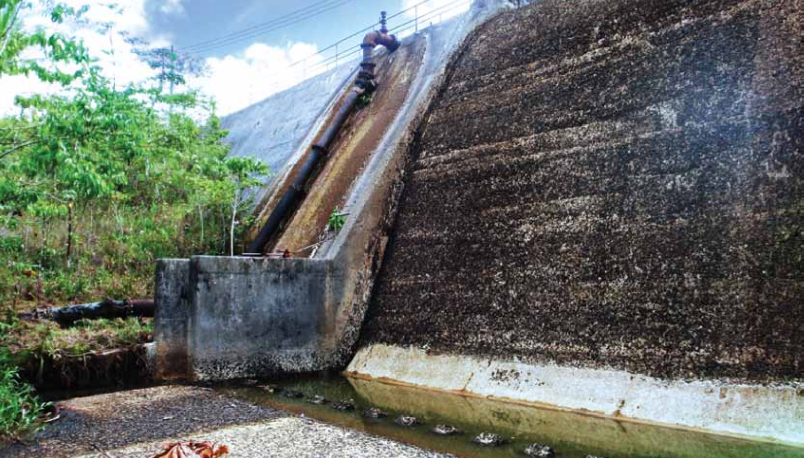
Ngerimel Dam, water supply for Koror, Palau
