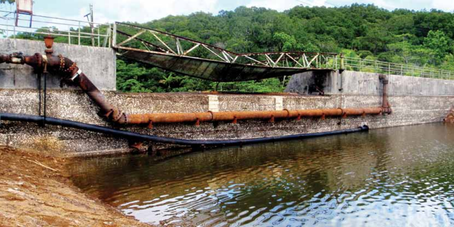
Ngerimel Dam, water supply for Koror, Palau
