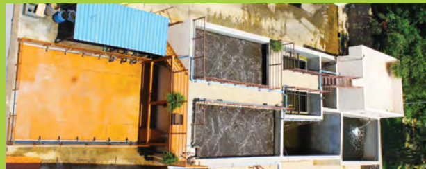
Waste Water Management
