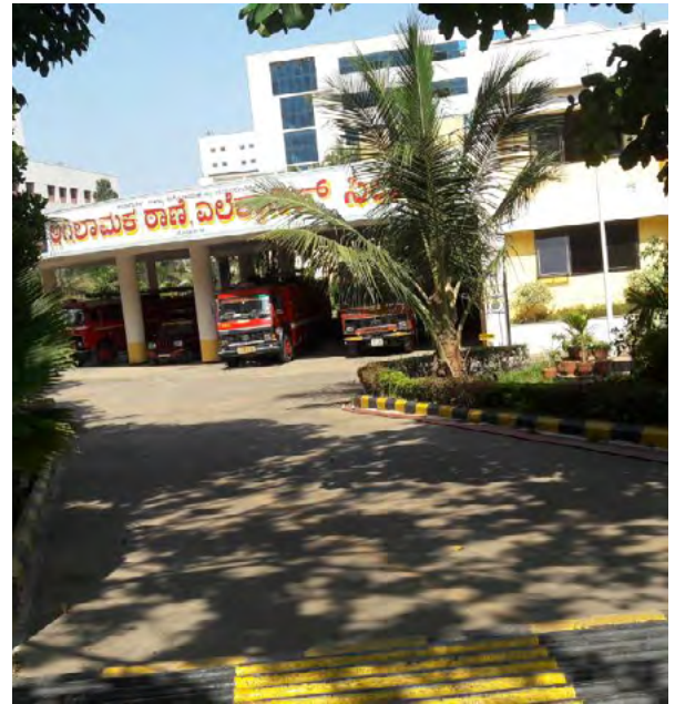
Electronics City has a fire station in the West Phase.
