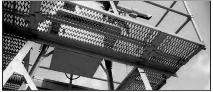
GRIP STRUT® is slip-resistant in all directions.
