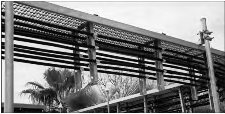
The serrated diamonds on GRIP STRUT® grating provide a safe walking surface for workers.
