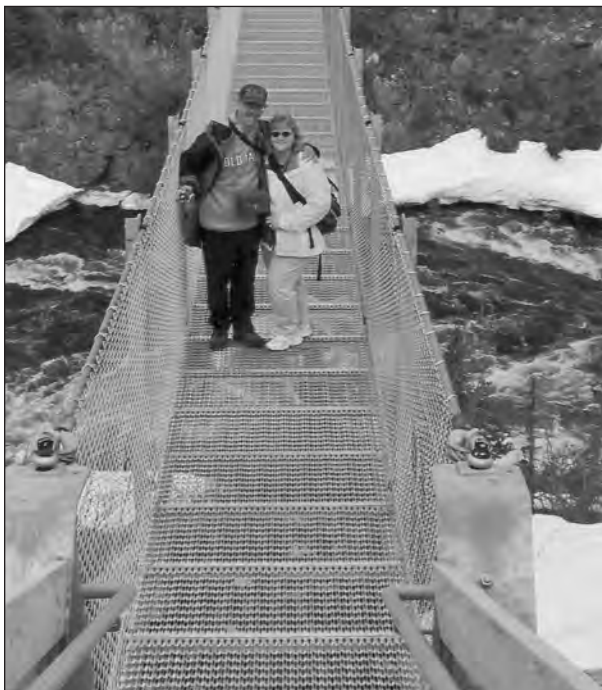
Safe, serrated GRIP STRUT® was used for this suspension bridge over the Canadian Tutshi River and Canyon.
