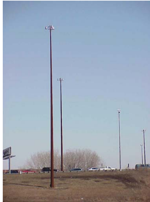
High Mast Tower Poles (3-100, 4-100, etc.)
