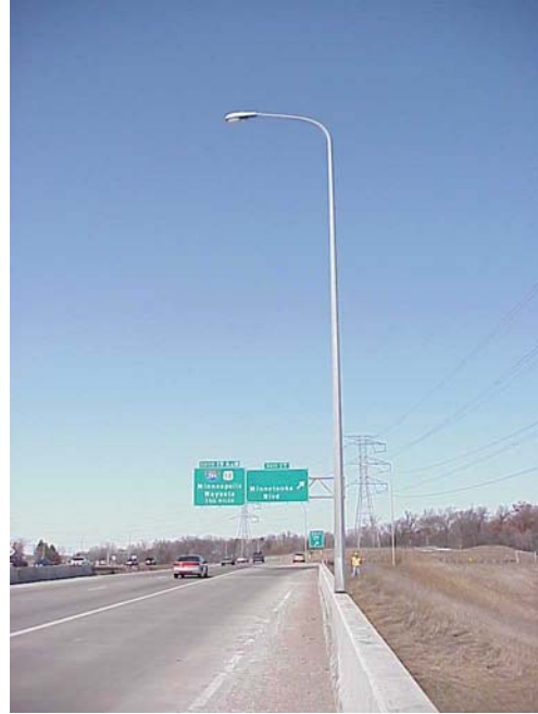
Bridge Pole (6B-40)
