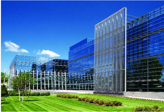
Global Research & Development Center, Suffern, NY.
