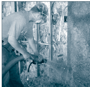
Damp-Blown Spray Cellulose Wall Insulation.
