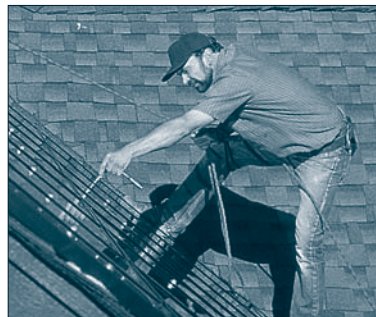
Installing Solar Water System.
