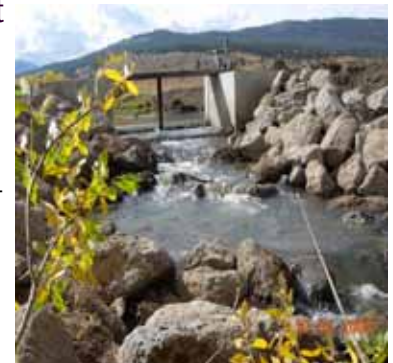
The new weir pays off with passage of Yellowstone cutthroat assured.
