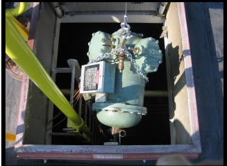
For use with "Cranky" Portable Winch. Simply set "Port-A-Post" on ladder and place "Cranky" on post. Quickly & securely sets on the roof hatch ladder or other permanent vertical ladder allowing the technician to easily lift heavy objects such as compressors and motors directly through the roof hatch or up a vertical ladder. Post includes double clipped rope for toting "Port-A-Post" & "Cranky" to roof in one trip. Slips on in approximately sixty seconds.
