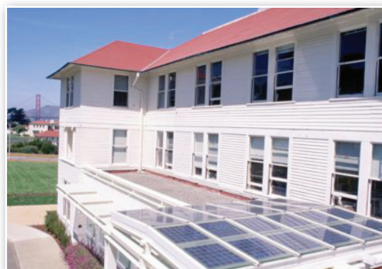
BIPV at historic Thoreau Center for Sustainability, San Francisco
