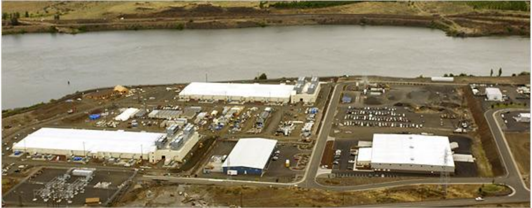
Google's data center on the Columbia river, Oregon
