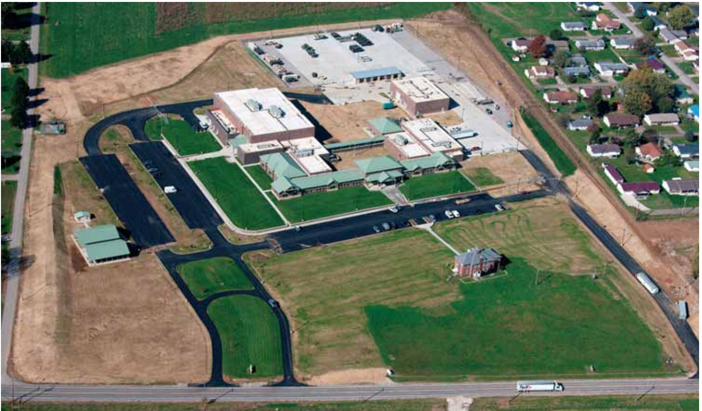
The $21 million Jackson County Armed Forces Reserve Center was opened on November 11, 2011, Veteran's Day. The 83,000-square-foot facility was built by Neighborgall Construction, Huntington, and designed by ZMM, Inc., Charleston. Photo by Mark's Photo, Ona.
