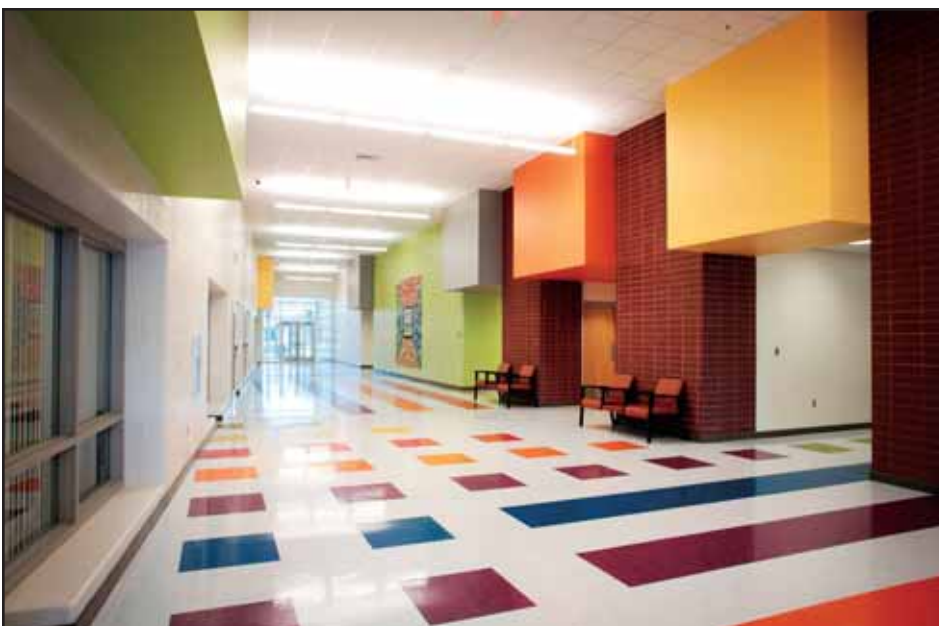
The West Side Elementary School, built by G&G Builders, Inc., Scott Depot, is the state's first totally integrated smart building. HVAC, security, fire and lighting systems all work in combination. Designed by ZMM, Inc., Charleston, the facility welcomed students for the 2011 school year.
