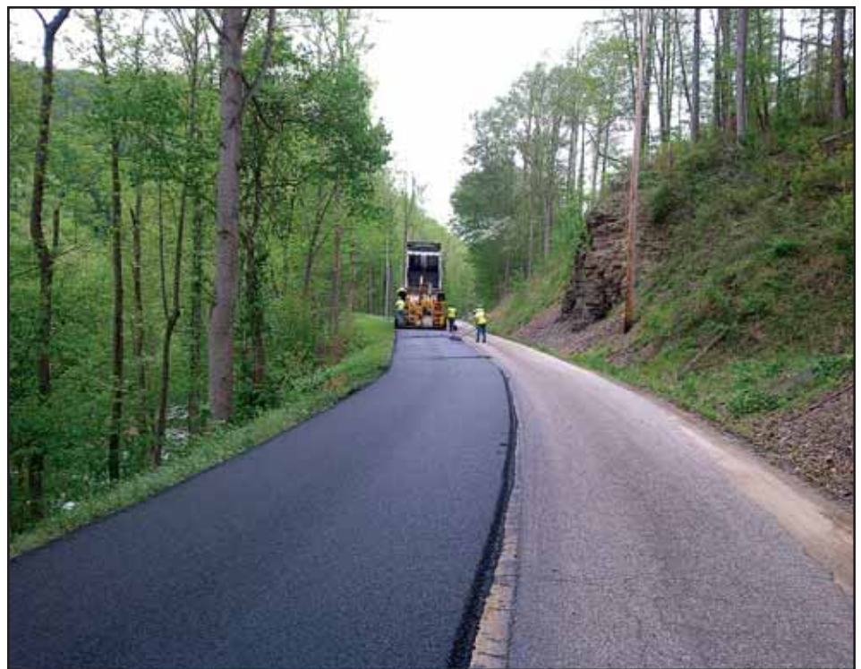
West Virginia Paving, Dunbar, lays Warm Mix Asphalt along a secondary road in Paint Creek in Kanawha County. The Secondary Road Paving Program received a funding boost in 2011. The 2012 budget includes $55 million for state contract paving, the same amount budgeted by the WV Division of Highways for 2011.
