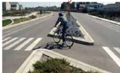
Median refuge island
