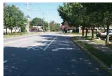
This intersection is properly striped; however, many are not or have faded markings.
