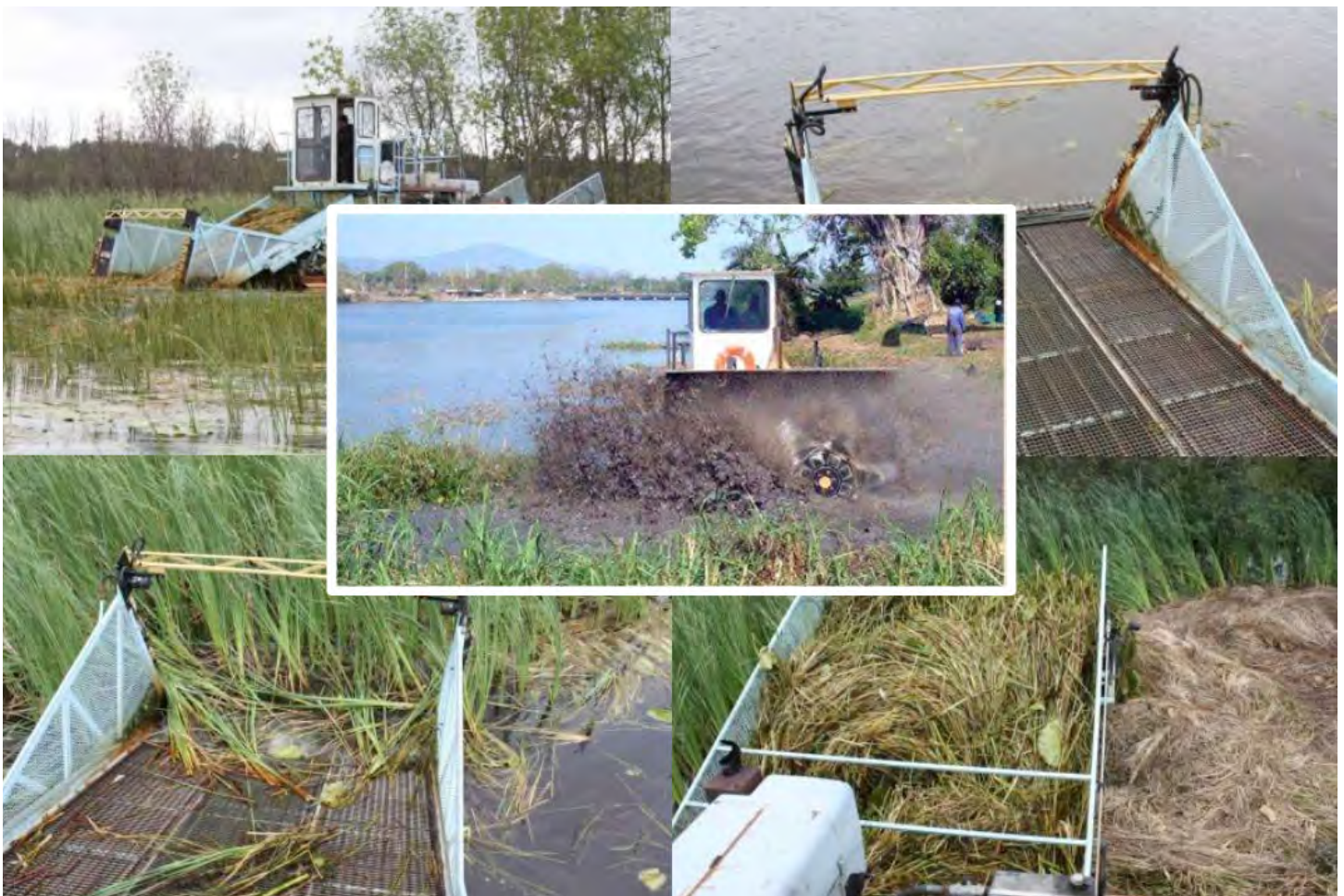
FIGURE 13. Floating cutter operating along Rainy Lake, Minnesota.
