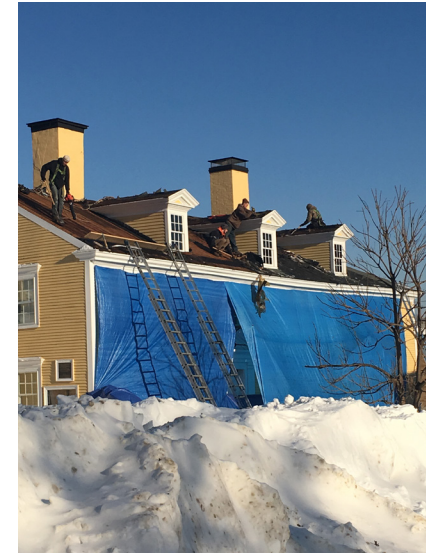
Roof installation at Ladd-Gilman House.
