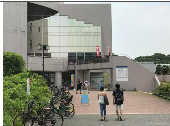
University Hall – Coop, Building S1-6. Cafeteria in the 2 nd Floor
