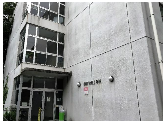
Building S6-3 Education and Cultural Hall near the main entrance (used on July 26 and 27 morning).
