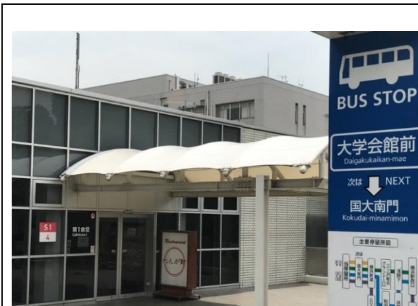
Cafeteria 1 Building S1-4 in front of Bus stop Daigakukan-mae (Near lecture room Bld S1-2)
