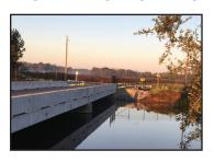
Constructed in 1965, this 140-foot timber-pile bridge over Mulligan Creek had undergone replacement and repair of its structural support timbers on two occasions over the years. When an annual South Carolina Department of Transportation inspection report recommended reducing the safe load capacity of the bridge to 10 tons, Beaufort County Council identified replacement of the bridge as a key project.
