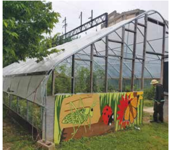
8th and Poplar Street Greenhouse prior to our team's renovations.
